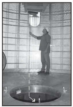
Photo 3-3 Broken arrow marks Metering Drum conduit installation under floor of walk-in cooling section and along inner wall of Hopper.
