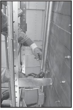
Photo 6-20 Clamping conduit to dryer.
