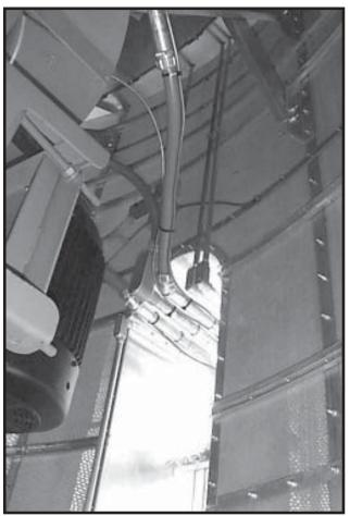
Photo 2-17 RH view - Fan Motors wired and Air Switch Tubing installed.
