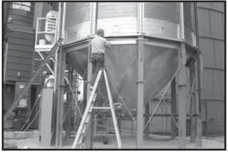
Photo 8-13 Running conduit for Fuel Train wiring.
