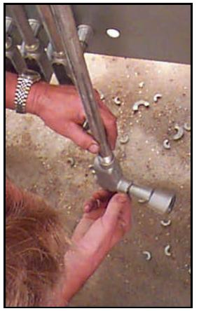
Weathertite Myers Hub -Photo B-3 portion installed to rear of Power Box (connects to portion inside Power Box).
