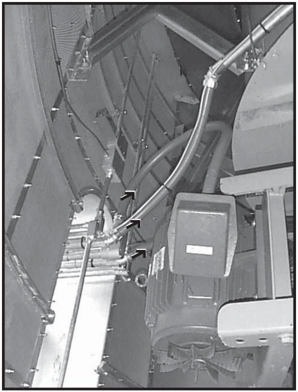
*Photo 2-2 Example: Wiring for (3) Fan Motors installed. Note 3/8" copper tubing for each air switch is wire tied to fan motor conduit. Note: fan cover is not yet installed.*
