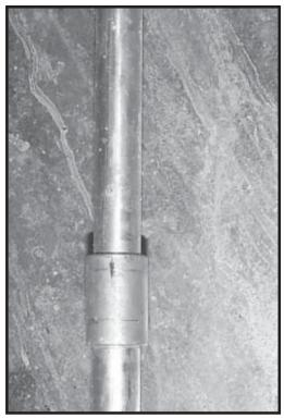
Photo 3-11 (B) Close Up - conduit coupling.
