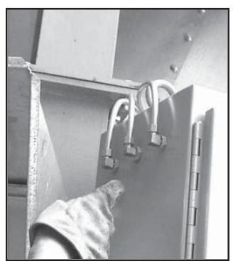
Photo 2-24 Brass connectors connect 3/8" copper tubing to Air Switches.
