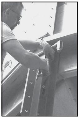
Photo 8-17 Putting Korn Clamp on conduit.
