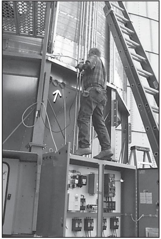
Photo 9-2 Installing lights and horn. Locate according to customer preference.
