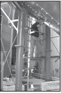
*Photo* 6-7 *Pulling wire for bindicator(s).*
