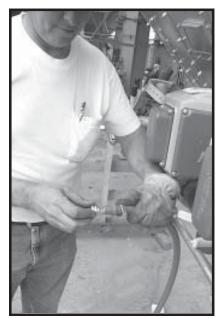
Photo 8-24 Attaching Sealtite fitting to Sealtite.
