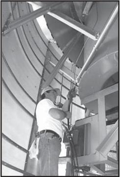
Photo 2-11 Drill hole in angle iron for mini clamp.
