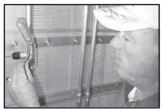
*Photo 4-7 Close Up - Conduit Tee in walk-in heating section with wiring and copper capillary.*
