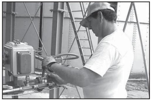
*Photo 8-26 Attaching Sealtite to conduit Tee from Modutrol Motor.*
