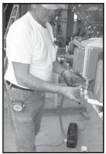
Photo 8-22 Attaching Sealtite to conduit Tee on Maxon Valve.
