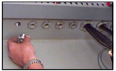
Photo B-2 Weathertite Myers Hub portion installed inside Power Box.
