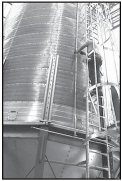
Photo 6-6 Installing Bindicator/Grain Temperature Sensor conduit.
