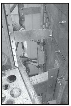
Photo 6-21 Threading conduit into Junction Box.
