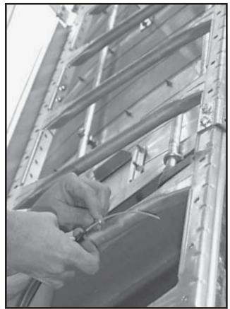
Photo 1-34 Tying wire to Fish Tape prior to pulling it through conduit.
