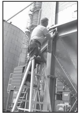
Photo 8-16 Installing LB-body.
