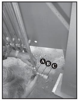
Photo 1-26 (A) LB-Body, (B) nipple, (C) exterior half of Myers Hub.
