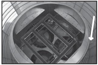
*Photo 7-4 Aerial view of burner with Ignitor and Flame Sensor conduit installed through burner housing.*
