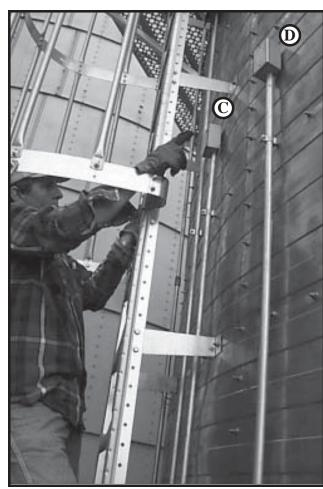
Photo 6-13 RH & LH Top Sensors (RTDs) installed.
