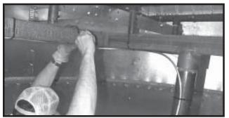
*Photo 8-8 Running 3/8" Pilot Fuel Line up along Burner Manifold to connecting point in Burner Pilot Section. Wire tie.*
