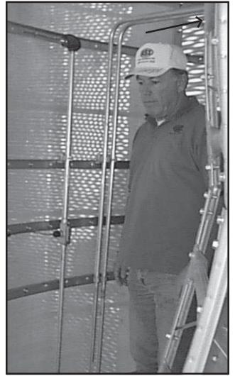
Photo 7-3 Run conduits up to level with bottom of burner.
