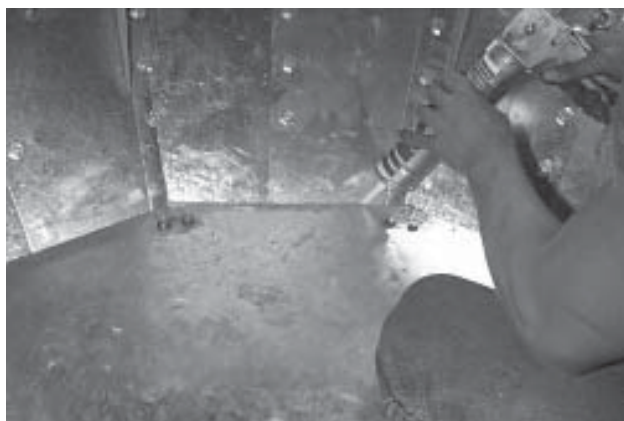
Photo 19-28 Caulking Metering Drum Floor with silicone caulk.
