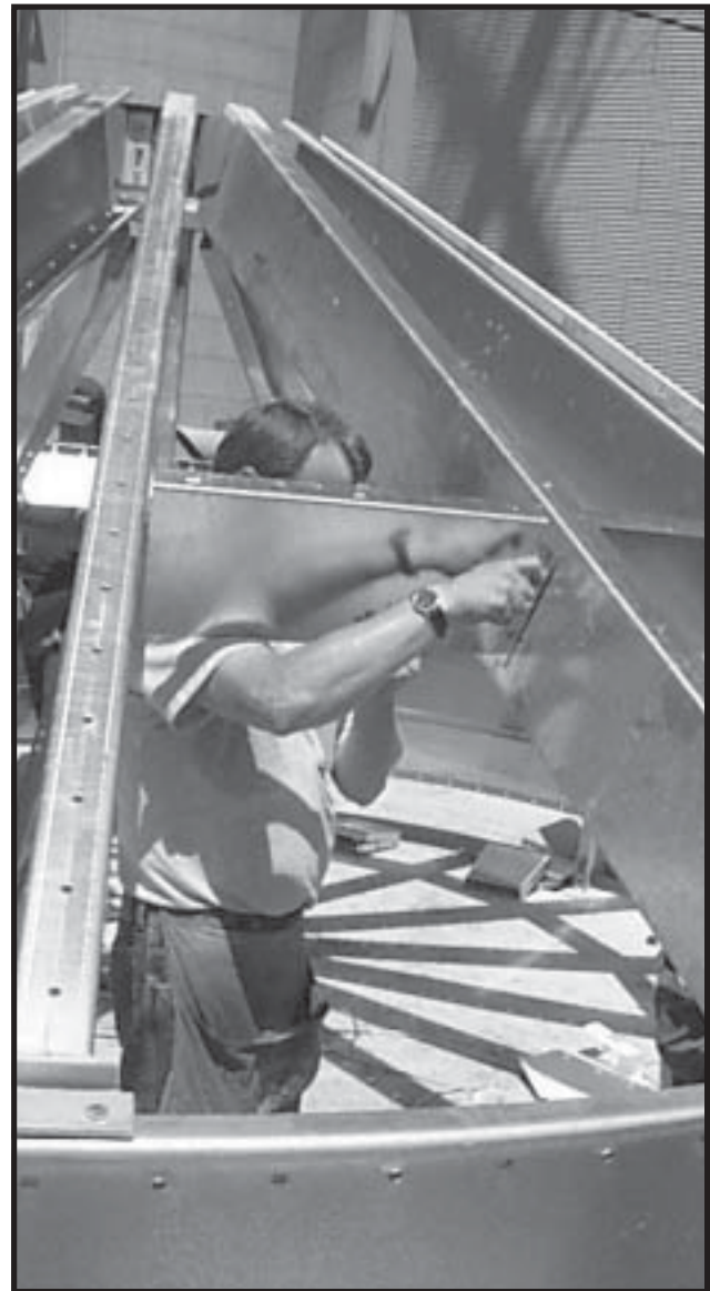
Photo 2-28 Installing Rafter CrossMembers.
