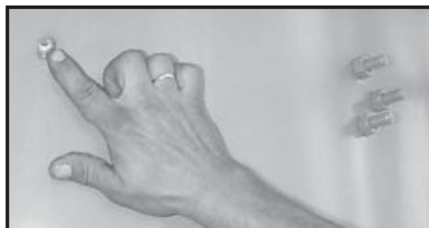
Photo 15-1 Close up - Grease Zert on Fan.
