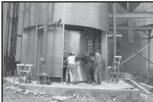
Photo 12-22 Move Reducer under Burner Housing.
