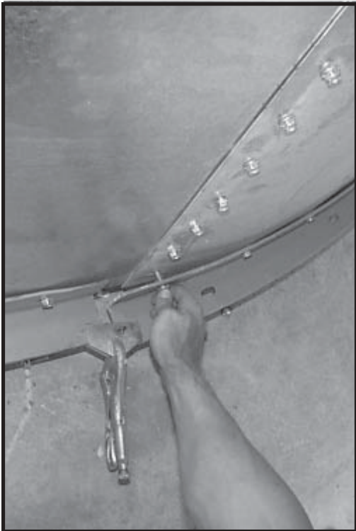
Photo 12-25 Close up - Bolting halves of Reducer Ring together.
