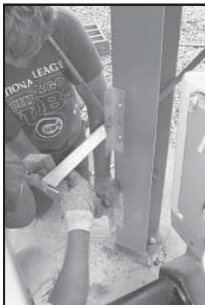
Photo 22-24 Close up - Bolting Fuel Train Stand.
