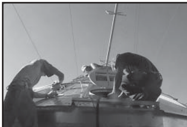
Photo 5-9 Installing Upper Bindicator.
