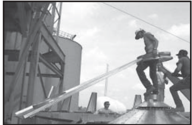
Photo 3-15 Bringing two opposing Tower Roof Sheets to Tower Roof Center Collar. Position Tower Roof Sheet with Access Port cutout directly above where outside ladder will be.
