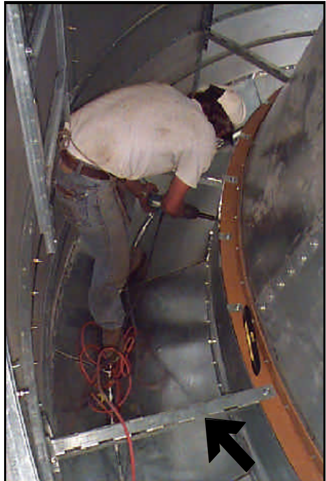
Photo 13-53 View from above Divider Hopper - Note: Wait to tighten Divider Hopper and Fan Skirting until after installing Reducer Walkway Support Beam (arrow).
