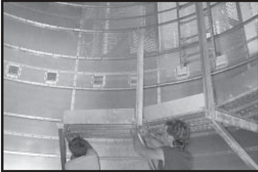
Photo 8-21 Installing Inside Catwalk.
