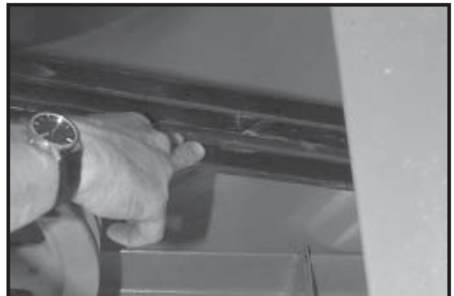
Photo 14-29 Checking Fan Belt tension. Can press down about one Fan Belt width.
