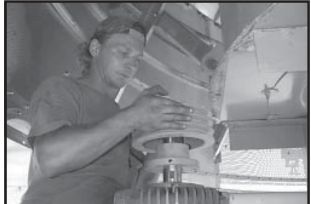
Photo 14-16 Sliding Motor Sheave on Motor Drive Shaft.
