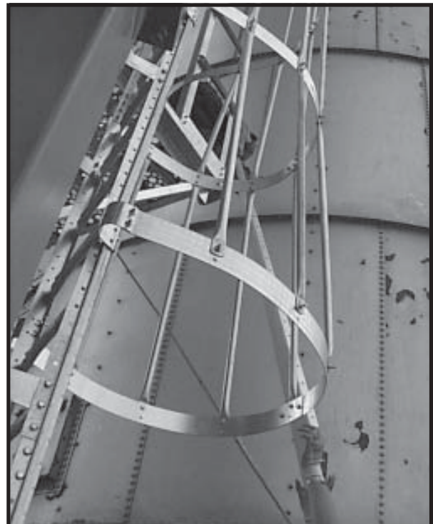
Photo 4-22 Bell Safety Cage installed.
