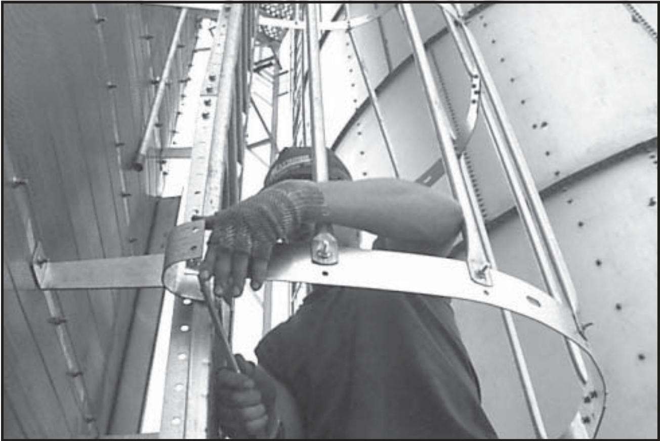
Photo 4-21 Close Up - installing Bell Safety Cage.
