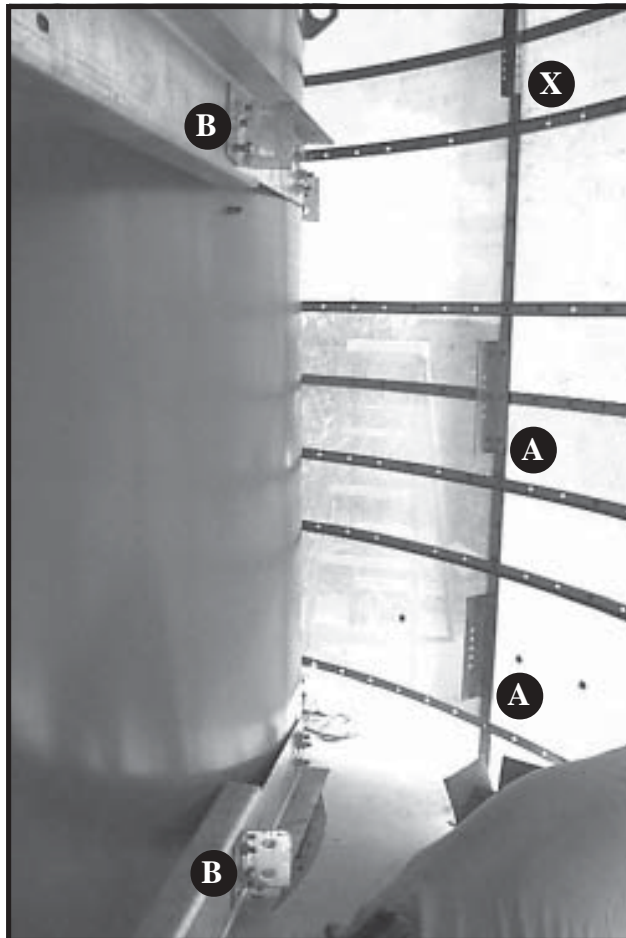
Photo 13-33 Clips installed.
