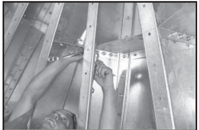
Photo 2-40 Hand tightening Rafter CrossMembers.
