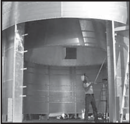
Photo 13-11 Checking clearance for Fan under Reducer/Burner.
