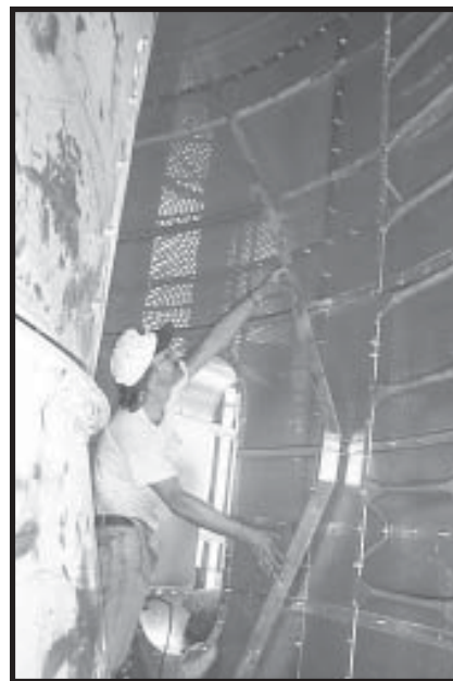
Photo 16-41 Installing 3" wide Heat Section Door Sleeve.
