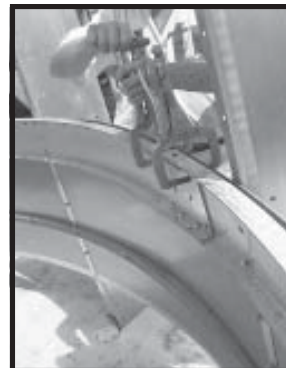
Photo 2-14 Splicing Plenum Eave Channels.
