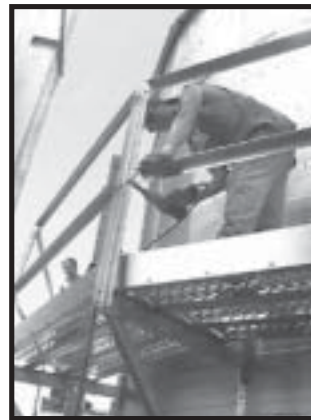
Photo 8-13 Tightening Outside Catwalk bottom Handrail.
