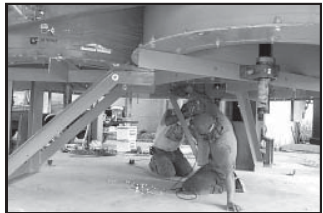
Photo 14-6 Tighting bolts on Fan Motor Mount.
