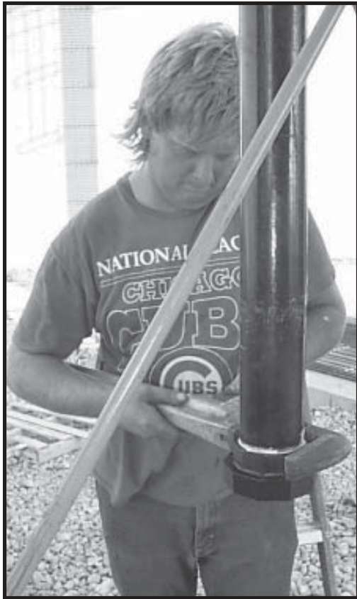
Photo 22-15 Attaching Union to Fuel Pipe.
