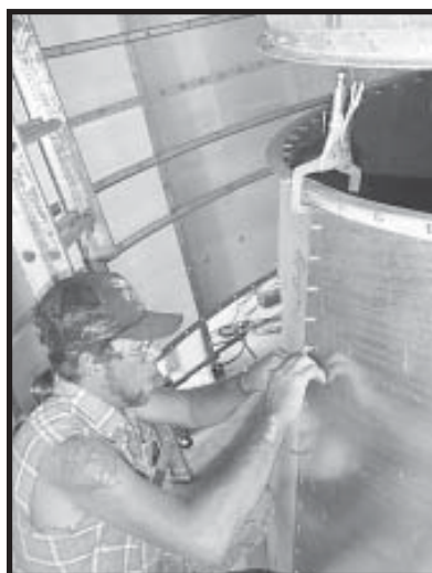
Photo 12-24 Bolting halves of Reducer together.
