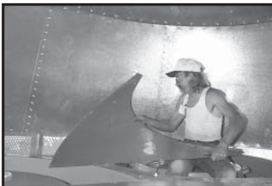
Photo 13-26 Positioning Fan Reducer Panel.
