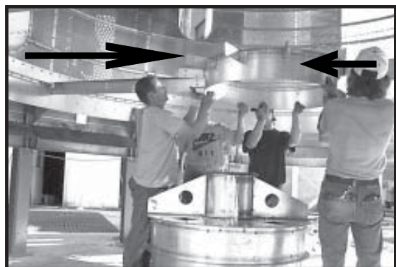
Photo 18-8 Bringing first pair of Cool Section Floor Beams (arrows) to Cool Section Floor Center Collar.
