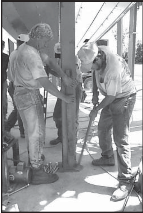
Photo 17-23 Tapping Dryer Legs into position.
