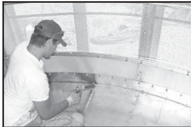
Photo 18-23 Caulking outside edge of Cool Section Floor.
