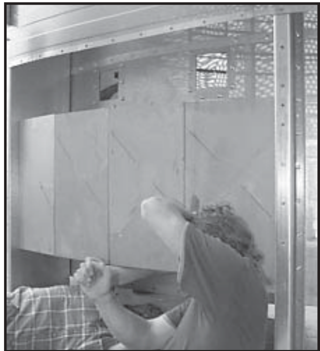
Photo 11-4 Installing middle Grain Turner Sections.
