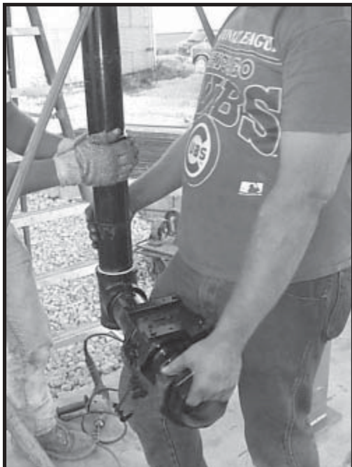
Photo 22-17 Connecting Modutrol Section to Fuel Pipe.
