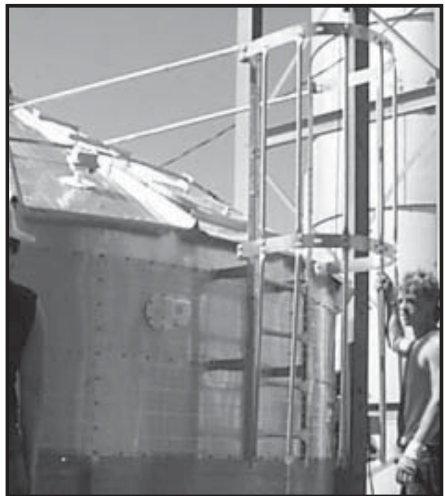
Photo 4-11 Installing Top Safety Cage to Tower Roof.
