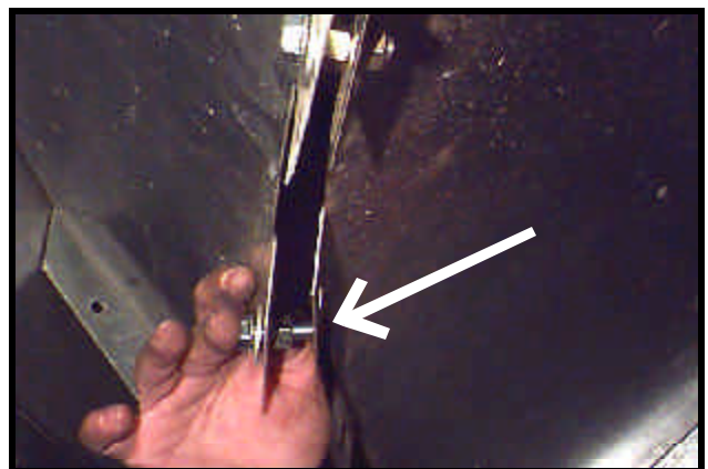
Photo 13-50 Close up - Using 3/8" nut (arrow) to space Outer Divider Hopper 1/4" from Inner Divider Hopper. Note: space between tabs will be 1/4" when outside nut is installed.
