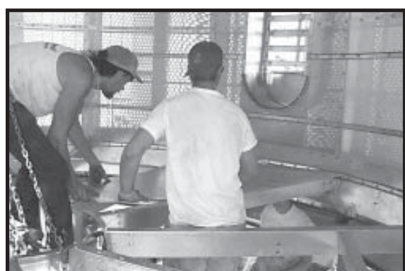
Photo 18-17 Placing Cool Section Floor Sheets.
