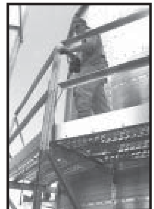
Photo 8-14 Tightening Outside Catwalk top Handrail.
