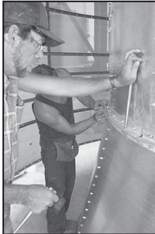
Photo 12-26 Aligning and bolting Reducer to Burner Housing.
