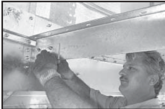
Photo 18-7 Snug bolting Cool Section Floor Beam to Cool Section Floor Beam Bracket (on Inside Solid Wall Sheet).
