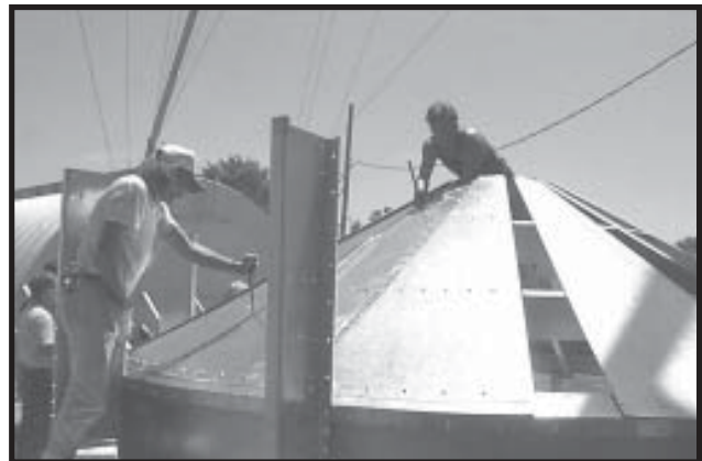
Photo 2-33 Aligning Plenum Roof Sheets.
