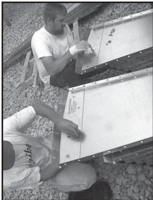
Photo 19-34 Pre-assembly (1) Inside Hopper Flange to each Inside Hopper Panel.
