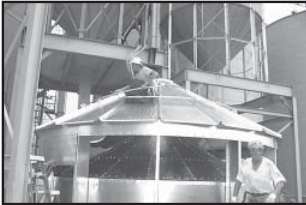
Photo 3-24 Installing Expansion Ring to Expansion Ring Clips.
