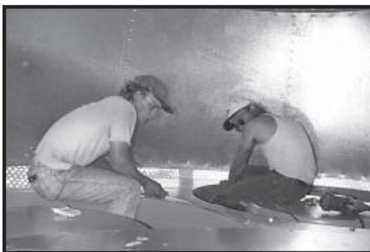
Photo 13-27 Bolting Fan Reducer Panel.
