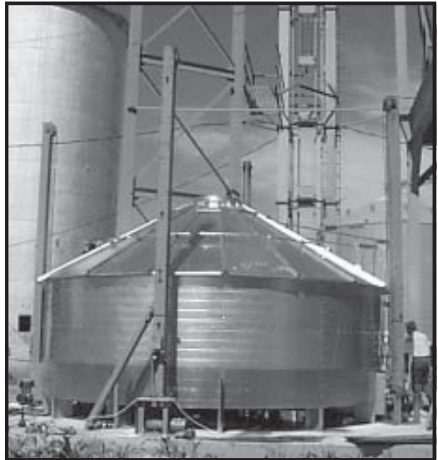
Photo 7-9 Jacks in place around dryer.
