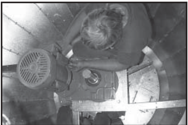
Photo 20-32 Bolting Motor to Gearbox (top mount). Note Motor to Gearbox configuration can vary.
