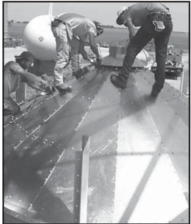
Photo 2-36 Installing Peak Cap to Plenum Roof Sheets.
