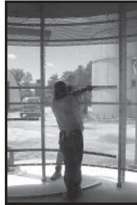
Photo 1-6 Installing Rolled Plenum Channels.
