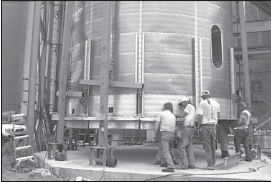
Photo 17-11 Compression Angle Weldments encircle base of dryer.
