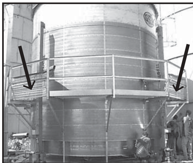
Photo 8-11 Catwalk installed with catwalk sections clamped where they will be installed after dryer is lifted clear of jacks.
