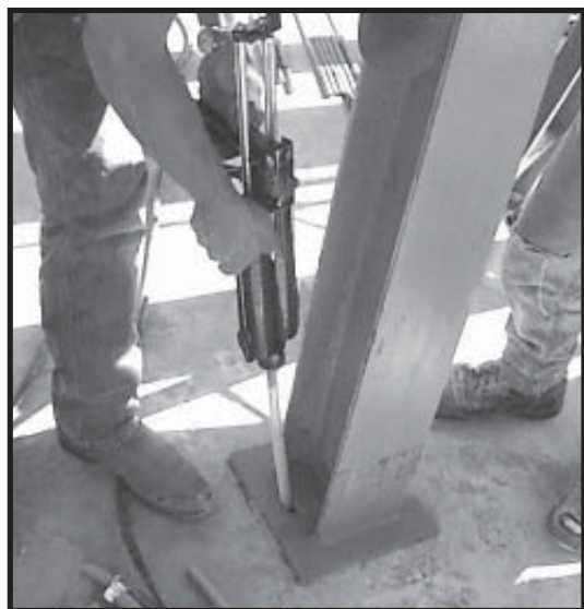
Photo 17-32 Fill hole with Ceramic Epoxy.
