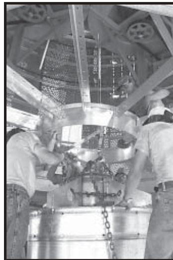
Photo 18-15 Securing Metering Drum for hoisting.
