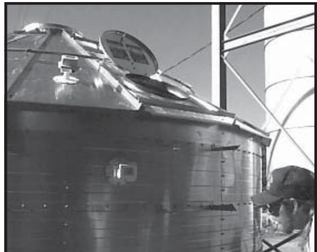
Outside View - access port installed with decals in place.
