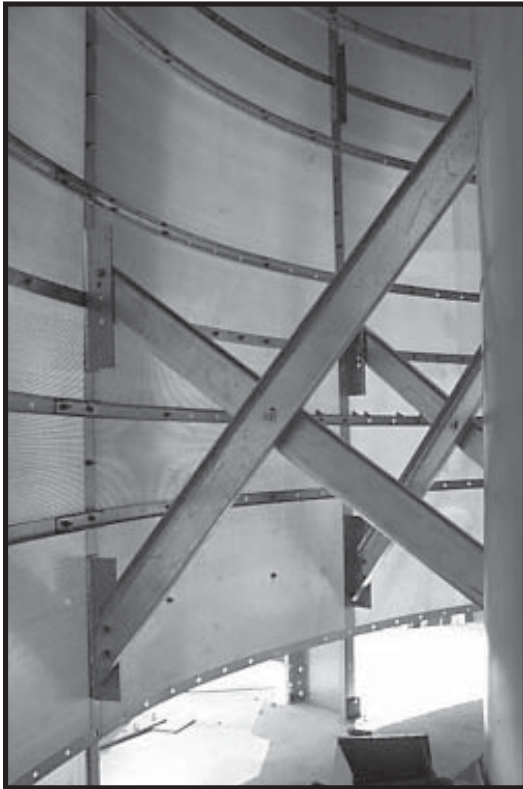
Photo 13-38 X-Bracing installed.
