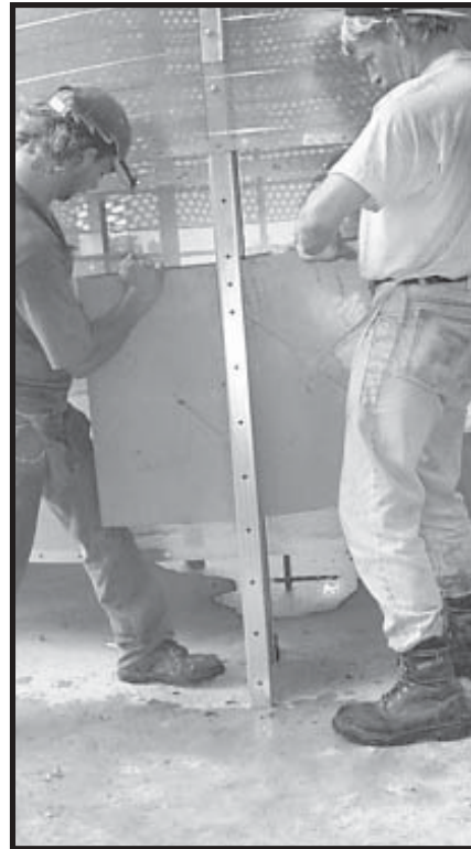
Photo 11-3 Installing outside Grain Turner Sections.
