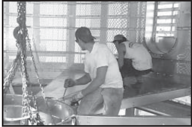
Photo 18-19 Aligning Cool Section Floor Sheets.
