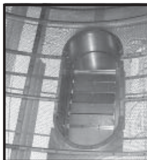
Photo 16-34 Installed 24” Louvered Window, with louvers closed.
