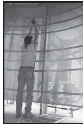
Photo 1-8 Tightening Inside Wall Sheets.
