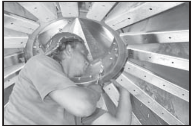
Photo 2-39 Hand tightening Plenum Roof Rafters.
