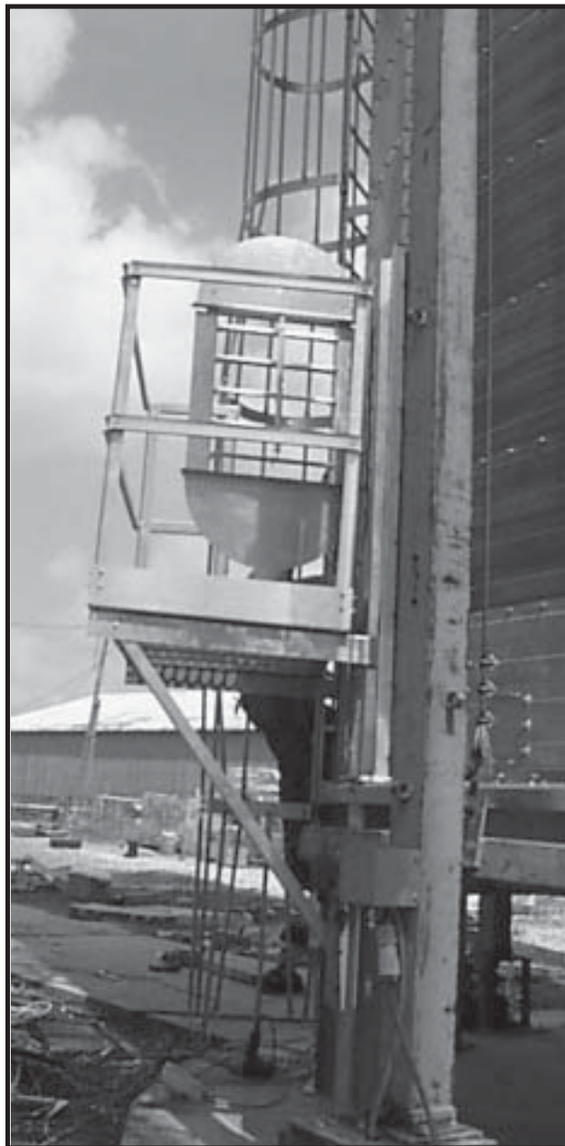
Photo 14-37 Cool Section Door is installed.
