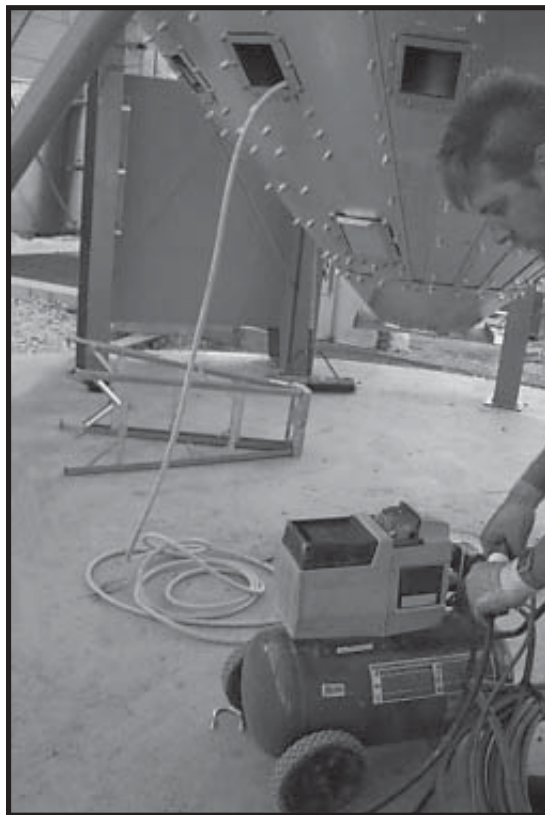
Photo 20-35 Filling Gearbox with Amoco Perma Gear 220 (or equivalent lubricant).
