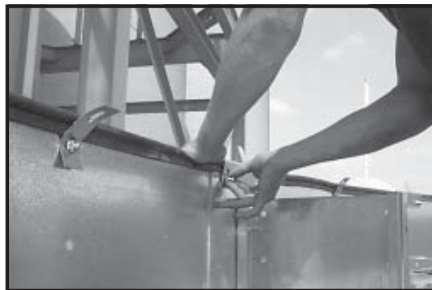
Photo3-8 Installing Eave Clip and Intermediate Eave Clips.
