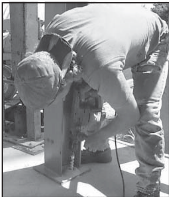
Photo 17-30 Drill proper size hole.
