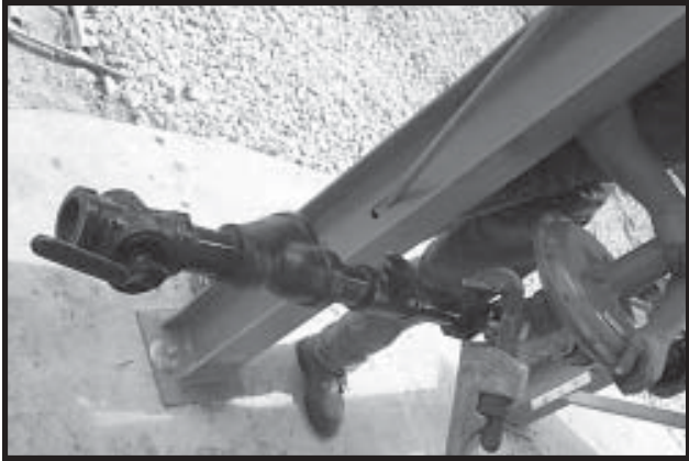
Photo 22-26 Installing Shutoff Section.
