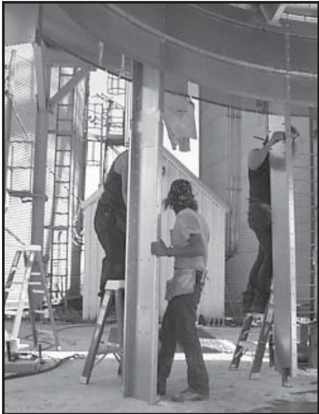
Photo 7-14 Close Up - Bolting Vertical Channels.
