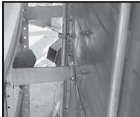
Photo 4-14 Close Up - Outside Ladder Brackets.
