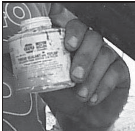
Photo 22-12 Seal all threaded pipe connections with Heavy Duty Pipe Sealing Compound.
