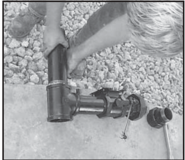
Photo 22-16 Attaching 12" Nipple to Modutrol Section.
