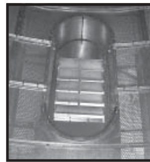
Photo 16-35 Installed 24” Louvered Window, with louvers open.
