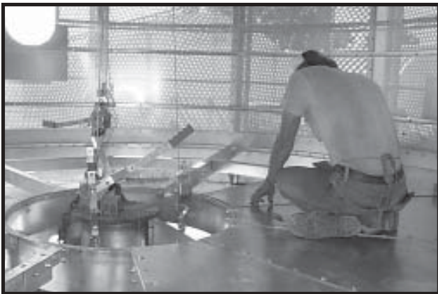
Photo 18-20 Snug bolting Cool Section Floor Sheets.
