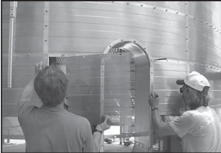
Photo 16-25 Fit Outside Wall Sheets to Window Frame.
