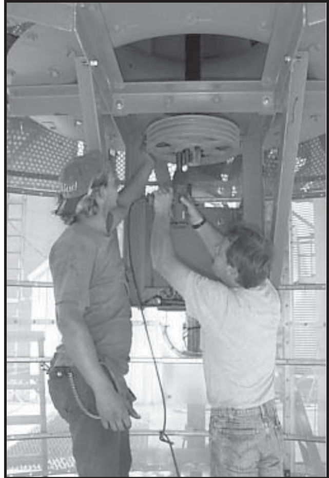
Photo 14-23 Tightening Fan Sheave bolts.
