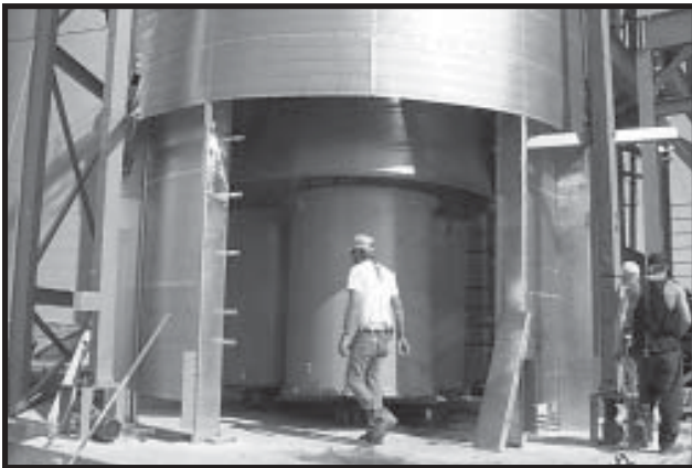
Photo 13-19 Three Fans form a cluster inside dryer.
