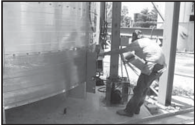
Photo 7-6 Positioning jack next to dryer.
