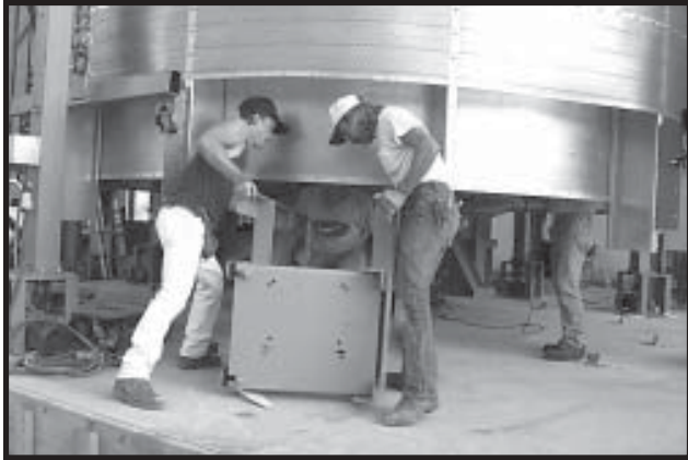
Photo 14-3 Moving Fan Motor Mount under Fan.
