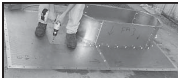
Photo 16-18 Bolt Window Frame to Wall Sheets.
