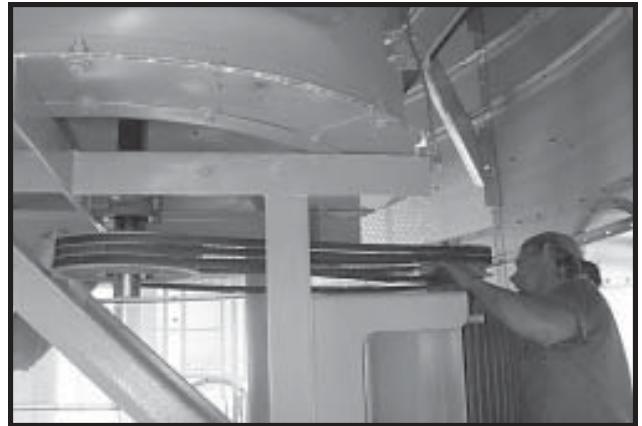
Photo 14-26 Running Fan Belts in grooves on sheaves.
