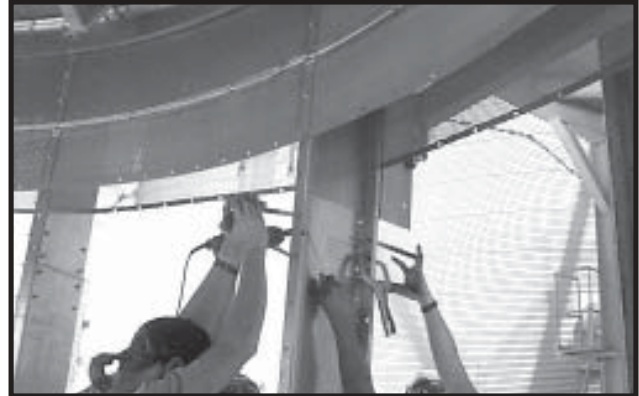
Photo 7-12 Aligning Vertical Channels.
