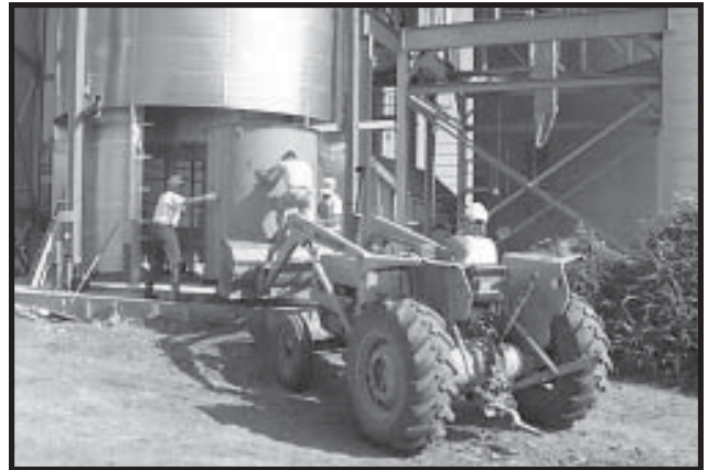
Photo 13-18 Pushing Fans into dryer.
