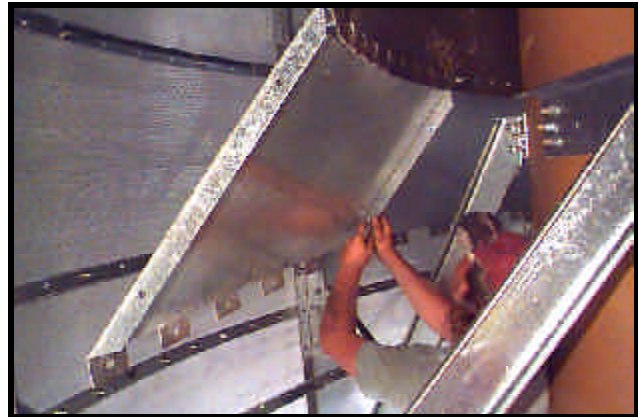
Photo 13-48 Bolting Inner Divider Hopper Sections together.
