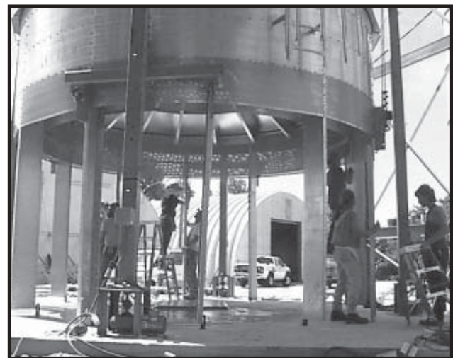
Photo 7-13 Bolting Vertical Channels.
