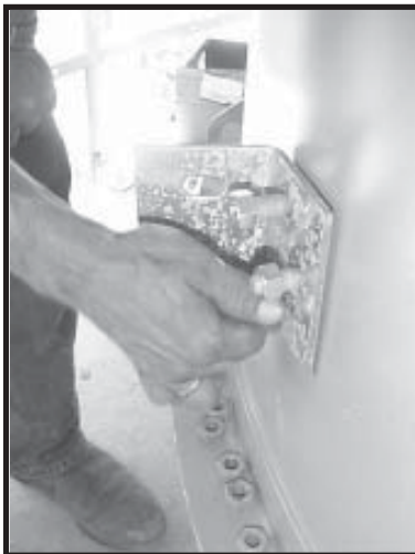
Photo 13-32 Installing Fan Cross Beam Clip to Fan.
