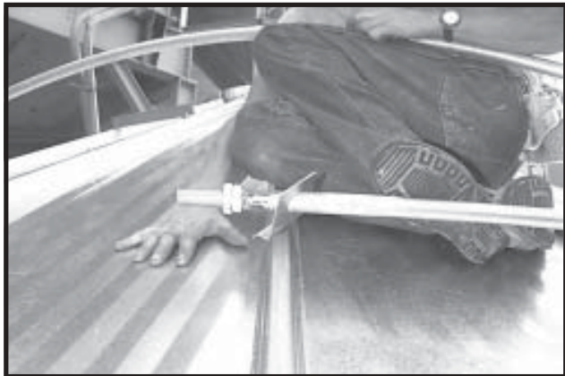
Photo 3-25 Close Up - Installing Expansion Ring & Clips.
