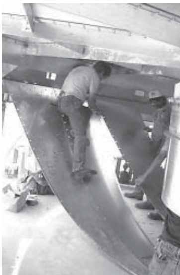
Photo 19-16 Aligning Outside Hopper Panels.
