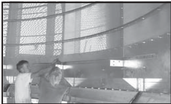
Photo 18-6 Installing last ring of Rolled Plenum Channel.
