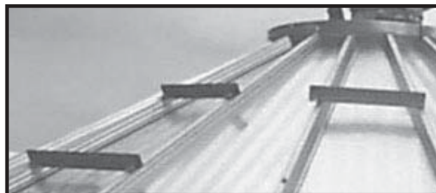
Photo 3-21 Close Up - Roof Rungs installed to ribs of Tower Roof Sheets.
