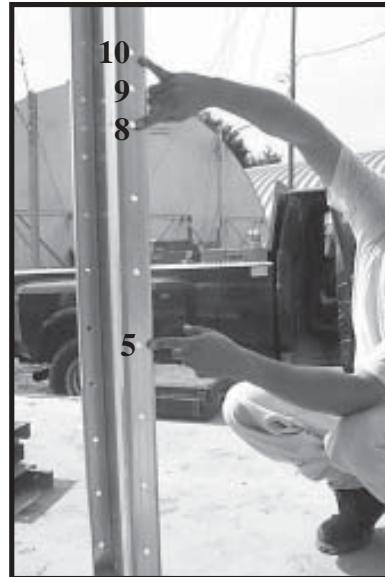
Photo 2-4 Do not fill bolt hole 5 (from bottom of Vertical Channel.) and 3 closely spaced bolts holes above, BH8, BH9, & BH10.
