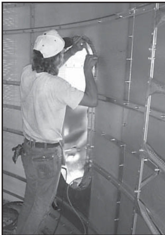
Photo 16-42 Wrapping Heat Section Door Sleeve around inside of Door Frame.
