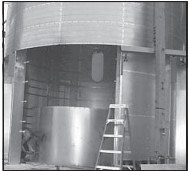
Photo 12-7 Bolting together halves of Burner Housing.
