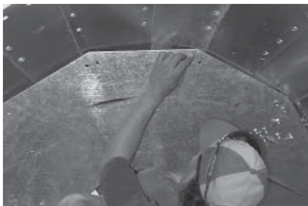
Photo 19-27 Close up - Installing Metering Drum Floor to Metering Drum Floor Clips.
