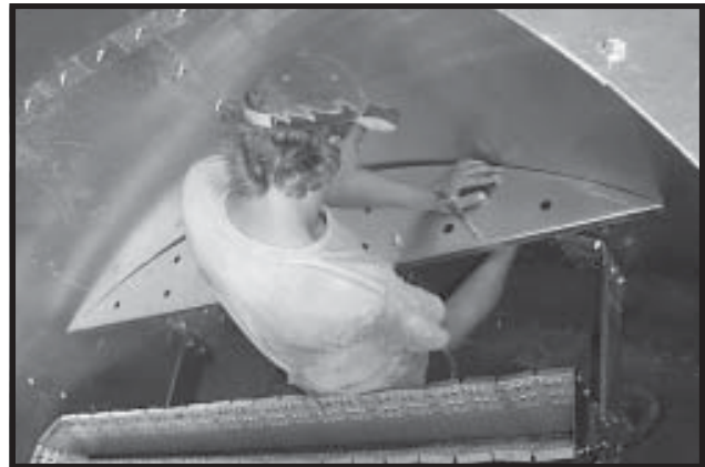
Photo 12-20 Installing Burner Baffles.
