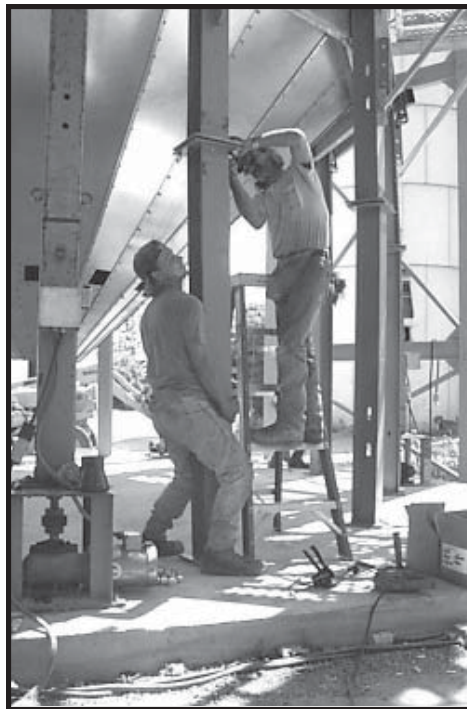
Photo 17-21 Bolting Lower Leg to Upper Leg.
