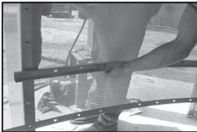
Photo 1-7 Close Up - Installing Rolled Plenum Channels.
