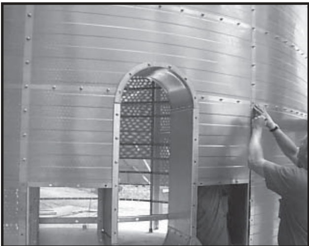
Photo 16-26 Bolt Outside Wall Sheets inside Window Frame.
