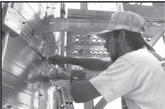
Photo 5-19 Installing copper capillary tubing with Insulated Clips.
