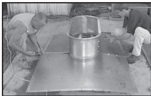
Photo 16-15 After cutting Window Outline, realign Window Frame to Wall Sheets and drill out bolt holes.
