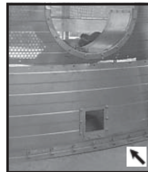
Photo 17-4 Sealing Strip (arrow) is installed to bottom of Outside Solid Wall Sheets.
