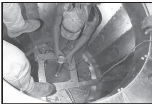
Photo 20-22 Sliding Gearbox Set Collar (2-3/8") onto Metering Drum Drive Shaft.
