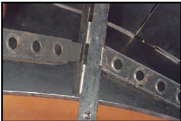
Photo 13-59 Close up - Inserting tab of Reducer Walkway Slat into slot on Reducer Walkway Support Beam.
