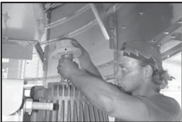
Photo 14-14 Sliding Motor Hub on Motor Drive Shaft.
