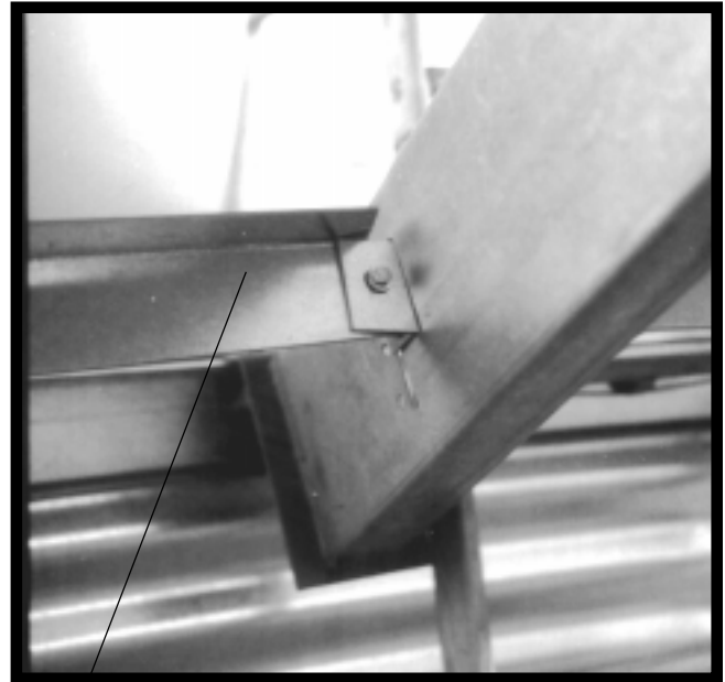
Floor Support Angle Assembly
