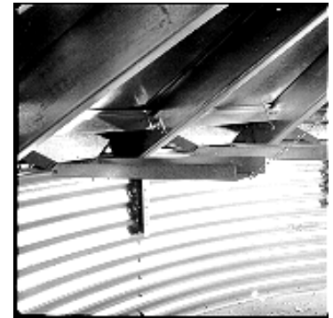
Chutes in closed position
