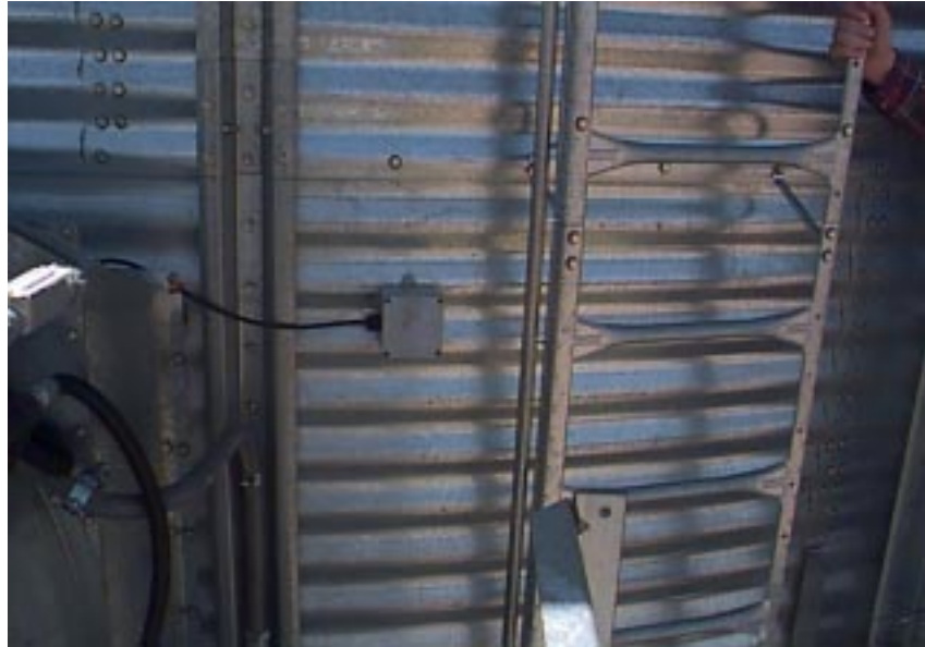
Plenum temperature sensor on the bin sidewall.
