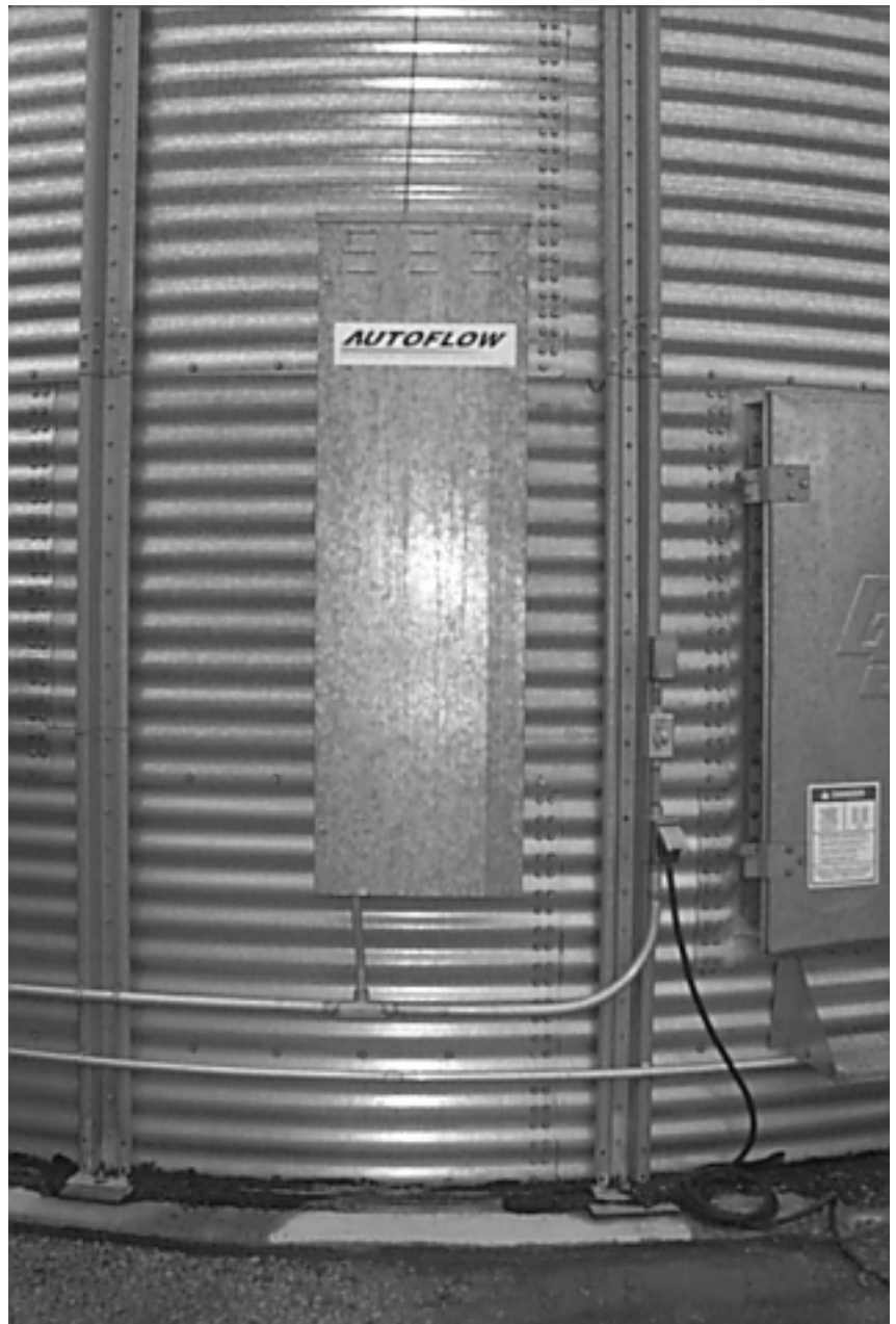
Actuator Control Box Mounted to Bin
