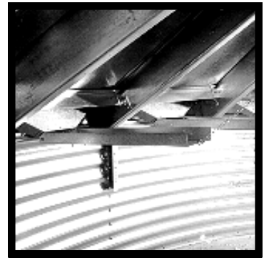
Chutes in closed position
