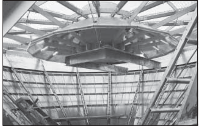
5-A. Bypass Gate During Assembly.
