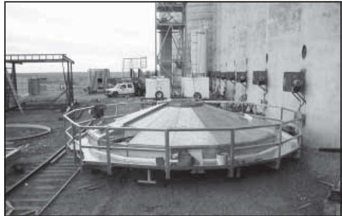
8-A. Platform during assembly. 50 KSS Shown.
