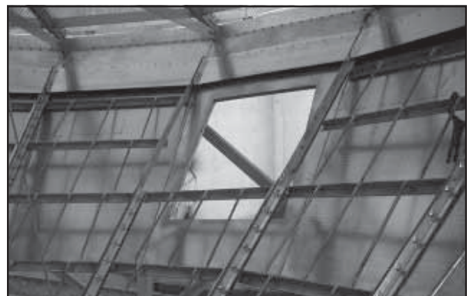
4-C. Installed Screen Frames on 50 K Scalper/Screeener.
