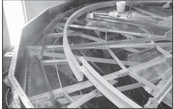
9-E. Drive Channel Halves During Installation.
