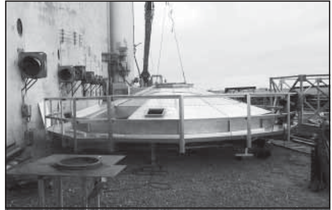
10-A. Top Shell during assembly.
