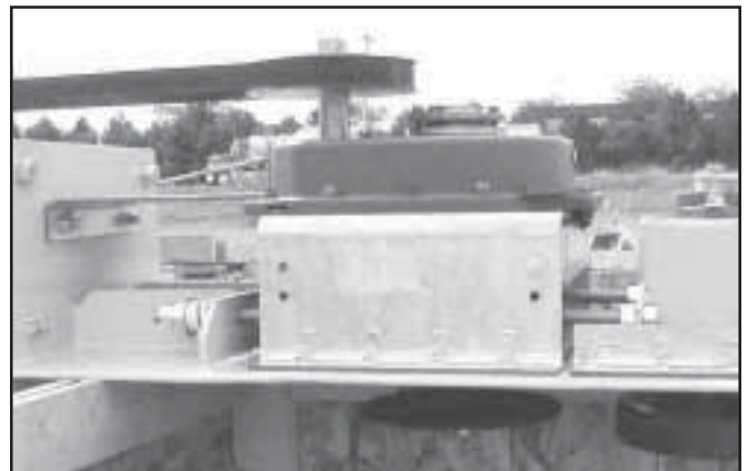
11-E. Drive shaft and sprocket installed.
