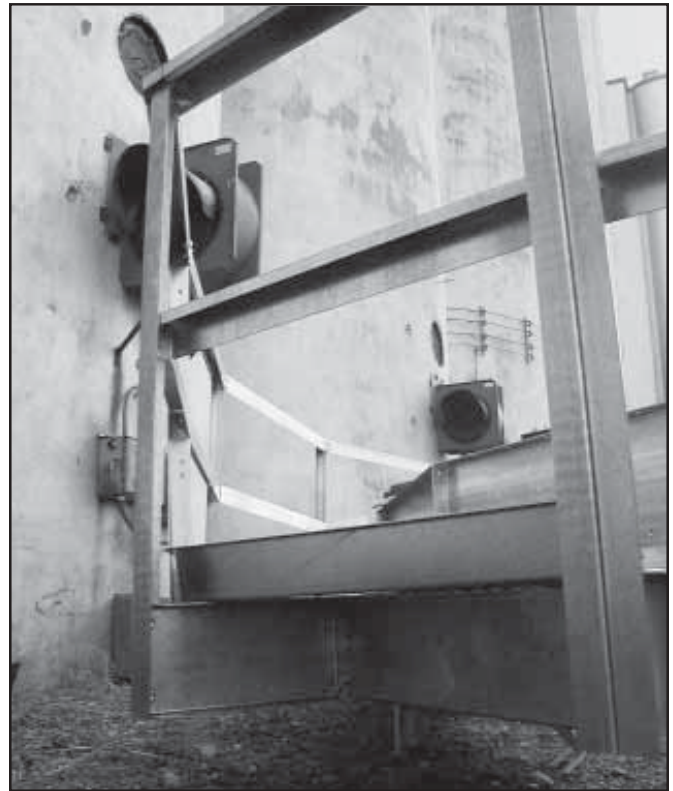
8-D. Platform Support Channels. RMS 15K Shown.
