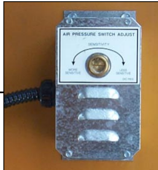
Air Switch assembly.
