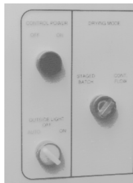
The work light switch can indicate a dryer shutdown.
