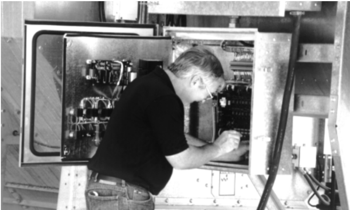
Airstream Service Technician checks the wiring on a dryer control panel.
