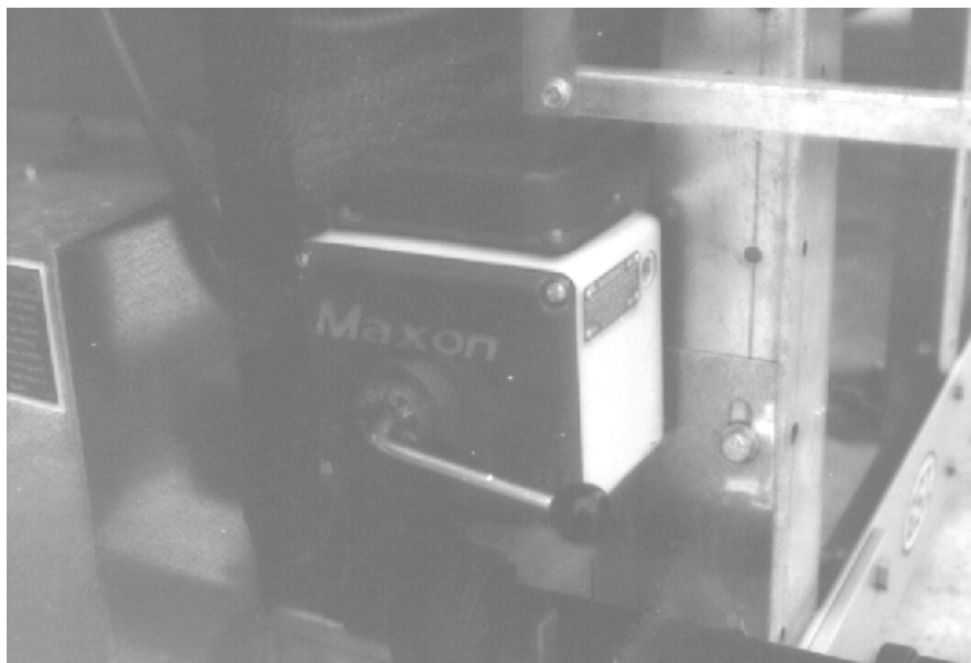
The Maxon safety shut off valve.
