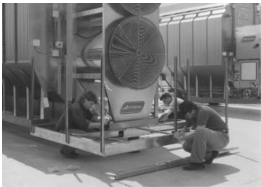
Figure 14: Install remaining support channels.
