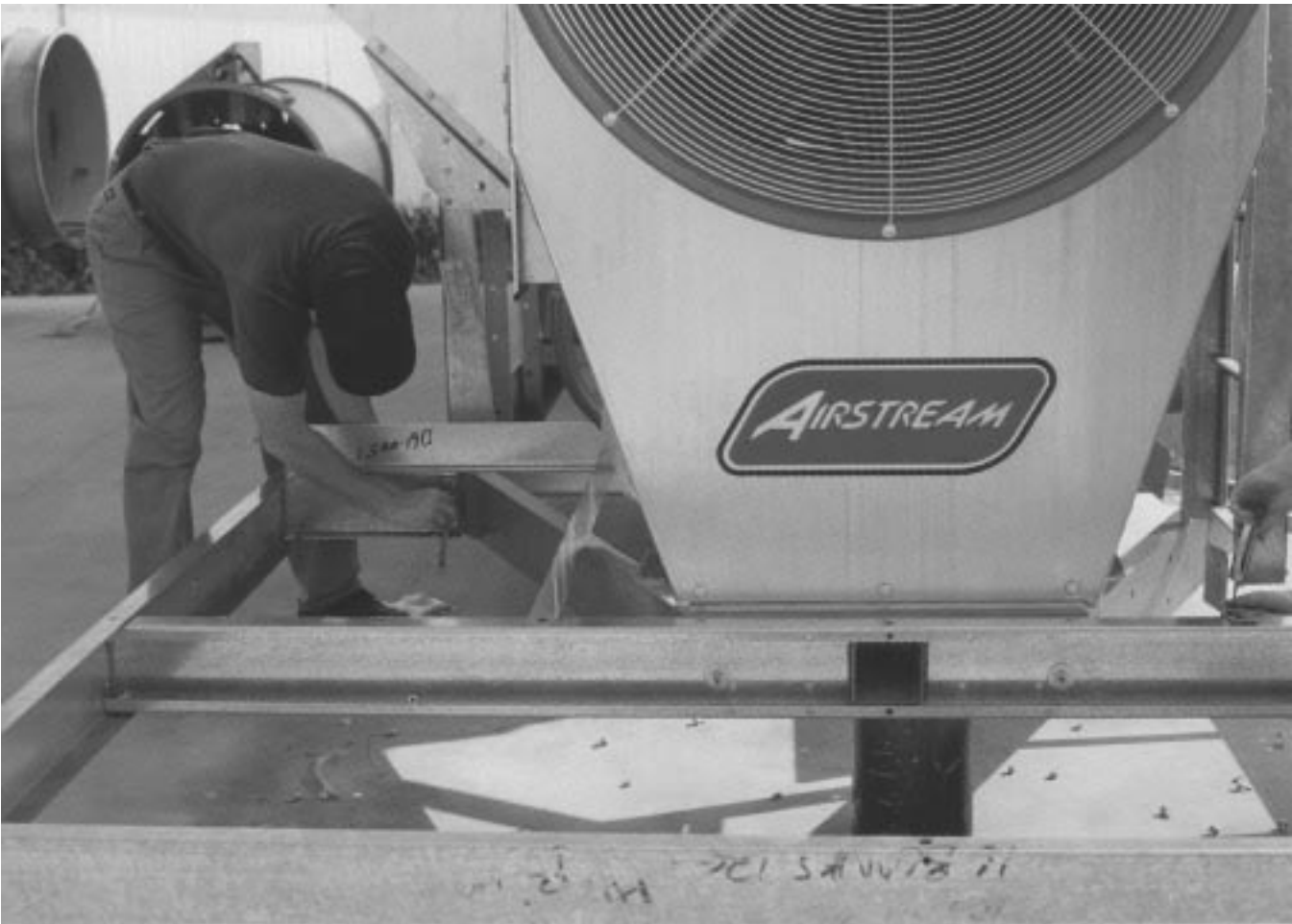
Figure 6: Tighten the rear frame tie angle to the side frame.
