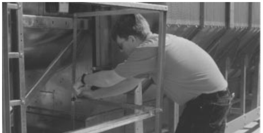
Figure 22, top: Installing front and side upper guard rails. Figure 23, above: Installing lower side guard rails. Figure 24, right: Installing lower rear guard rail.
