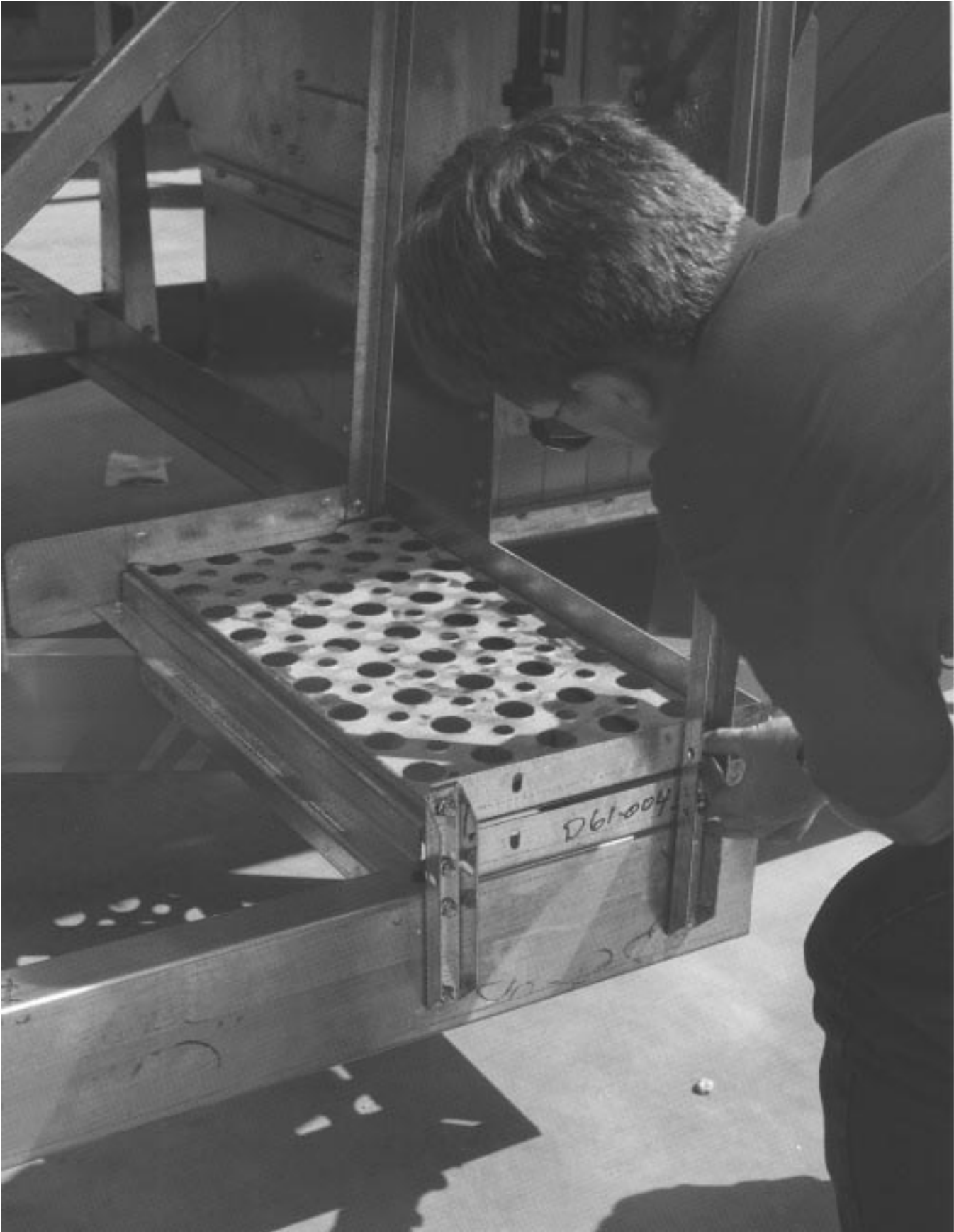
Figure 21: Installation of the short wide floor panel, left-hand outer rear toeboards and hinge channel.
