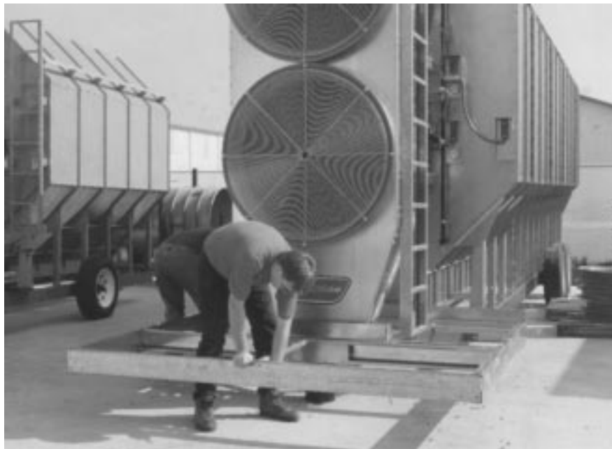
Figure 9: Center floor support placement.
