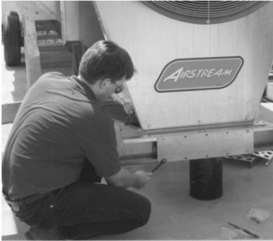
Figure 3: Bolting reinforcement plate to main support channel.
