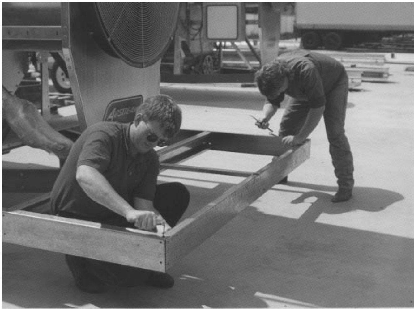
Figure 10: Check for square and tighten bolts.
