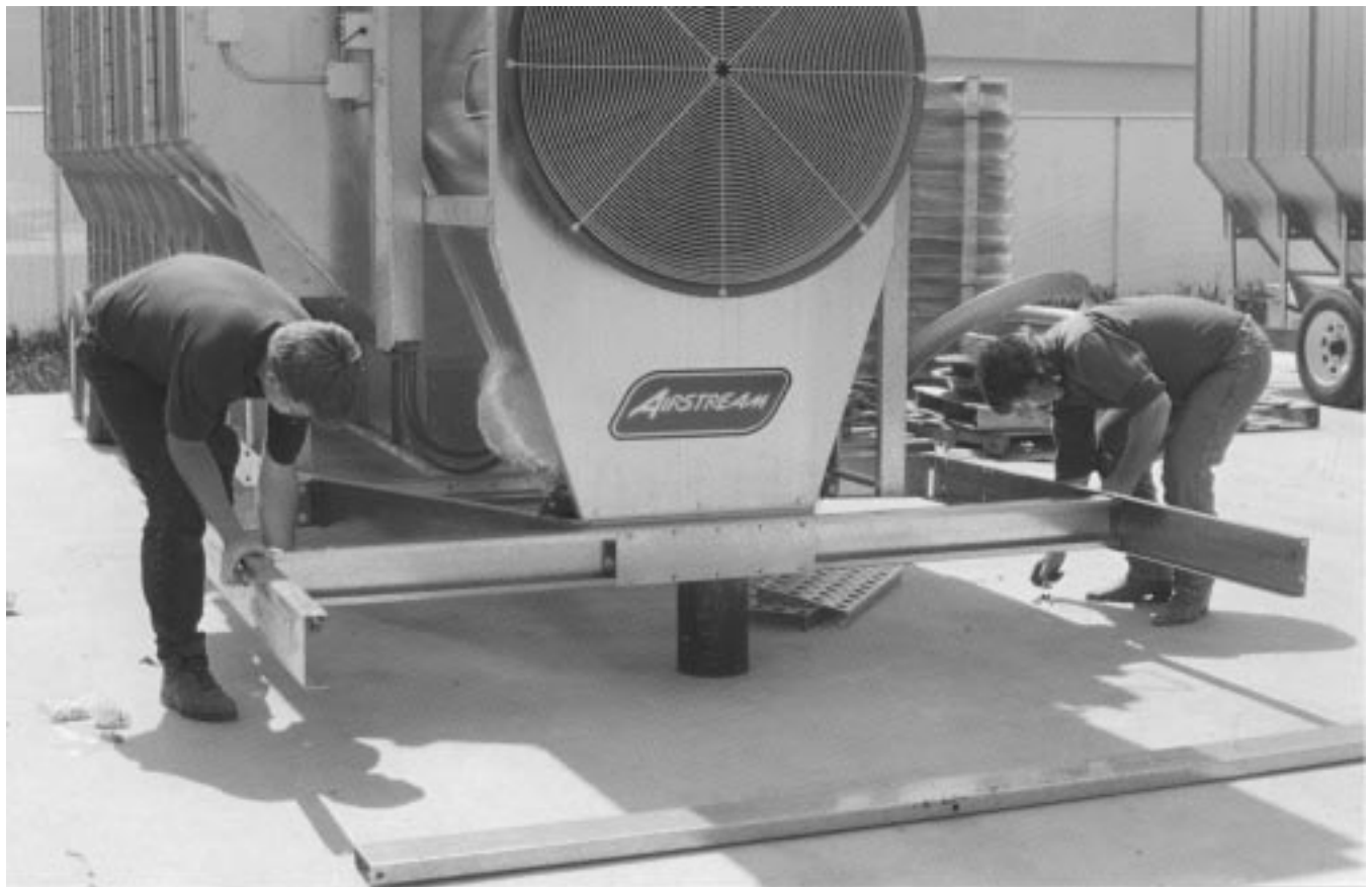
Figure 4: Attaching side channels.
