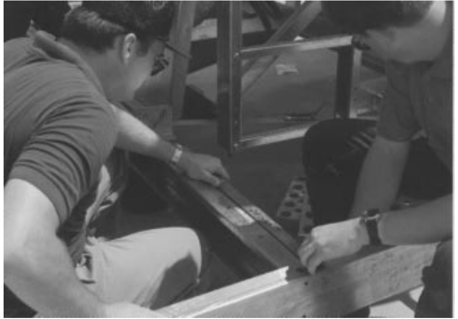
Figure 11: Installing forward frame on the access door.
