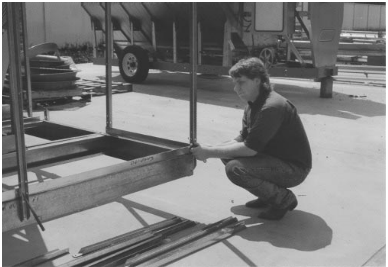
Figure 16: Connecting left-hand front toe board to guard rail support channel.
