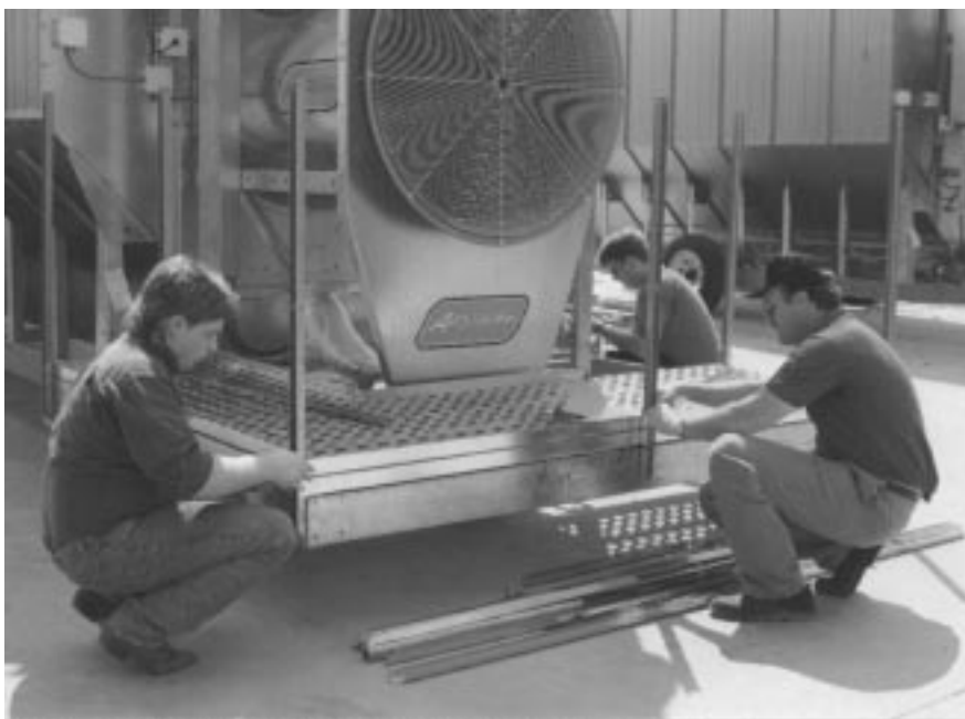
Figure 20: Installing the remaining toe boards.
