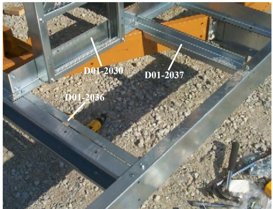
Figure 12: Close-up of forward and rear door frame installation.
