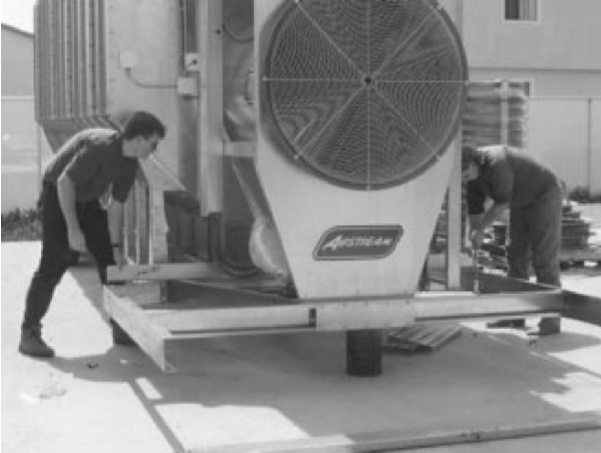
Figure 5: Placing rear tie angle on platform.
