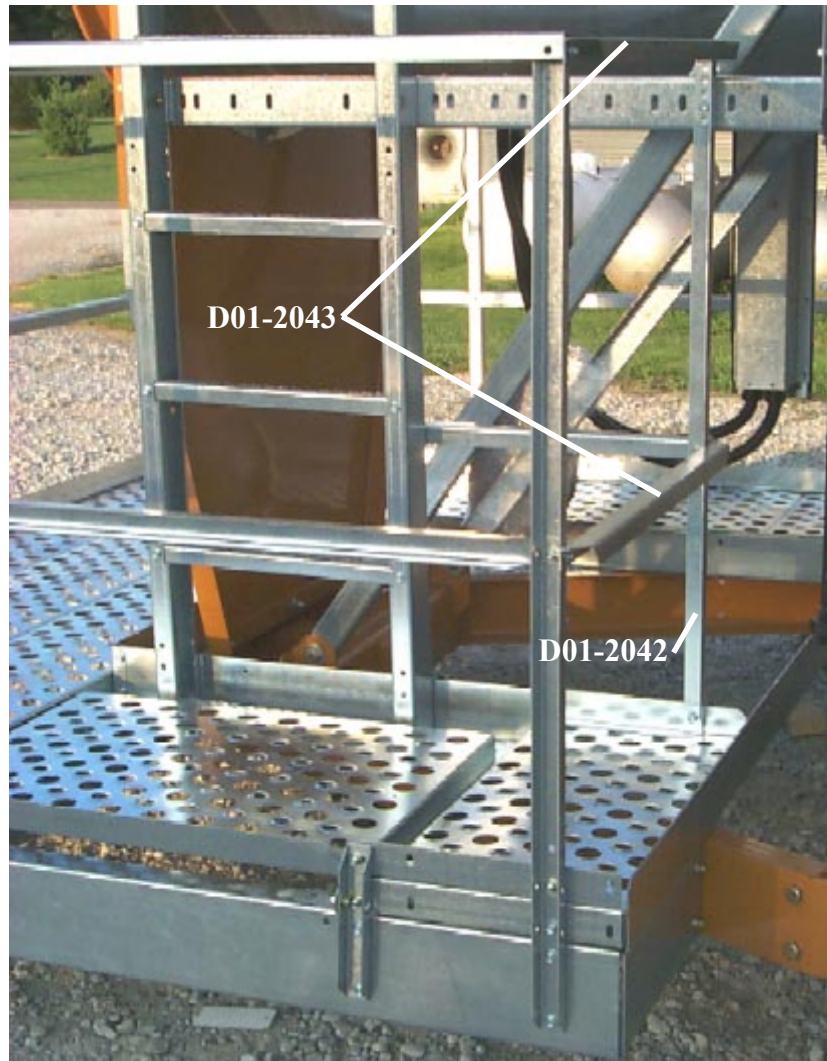
Figure 13: Location of inner guard rail support angles.
