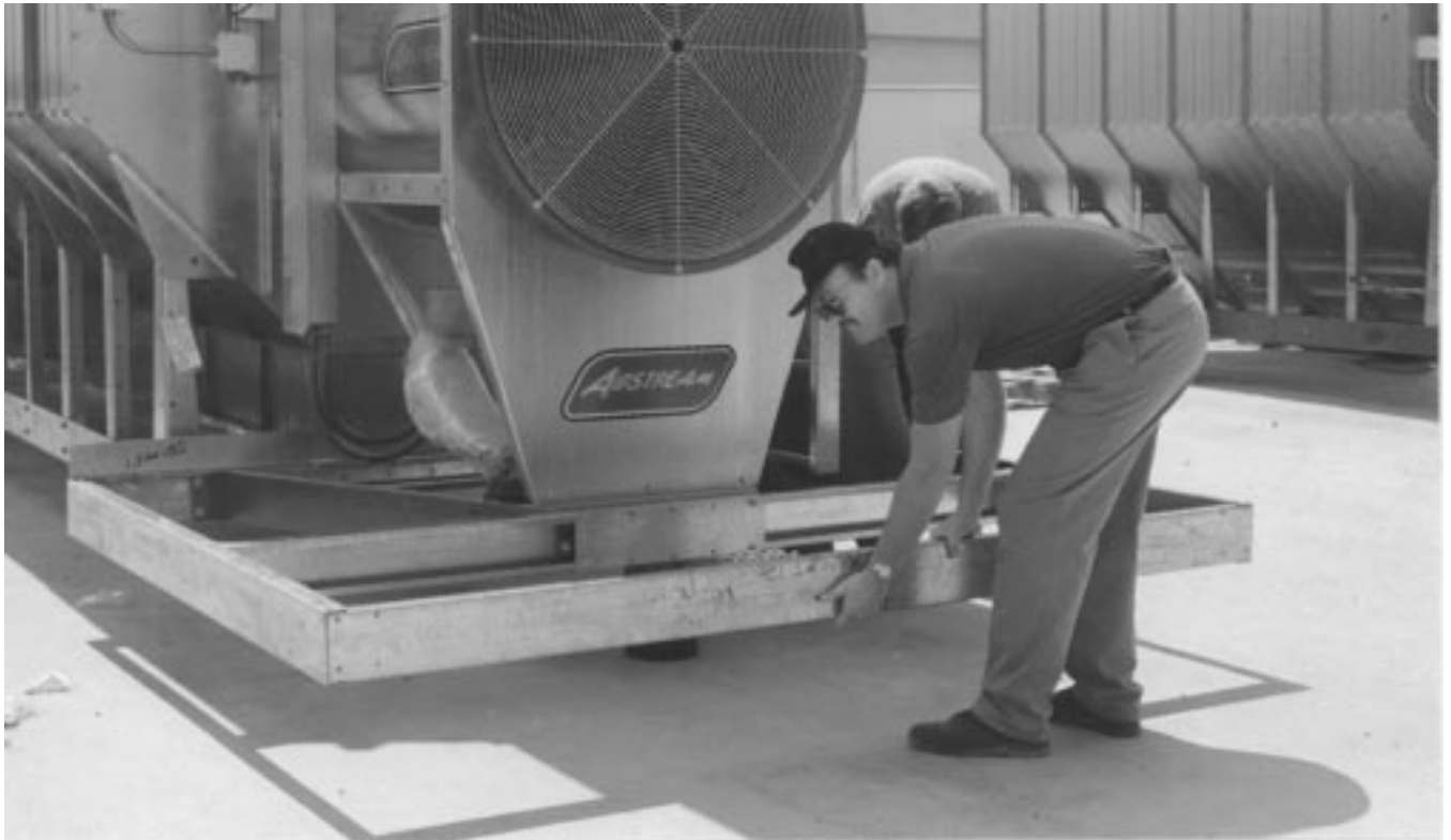
Figure 8: Attaching front channel.
