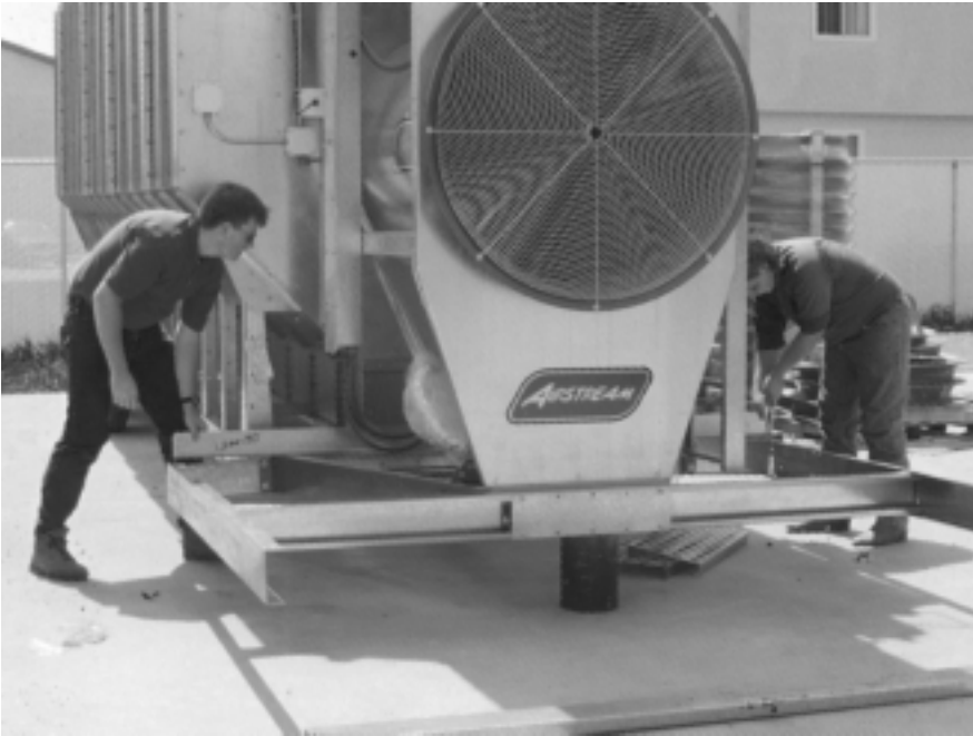
Figure 5: Placing rear tie angle on platform.
