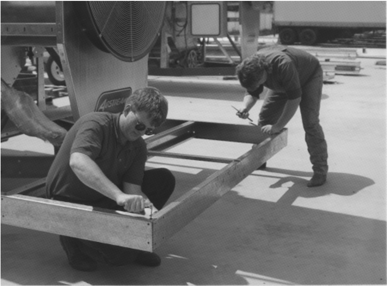
Figure 10: Check for square and tighten bolts.
