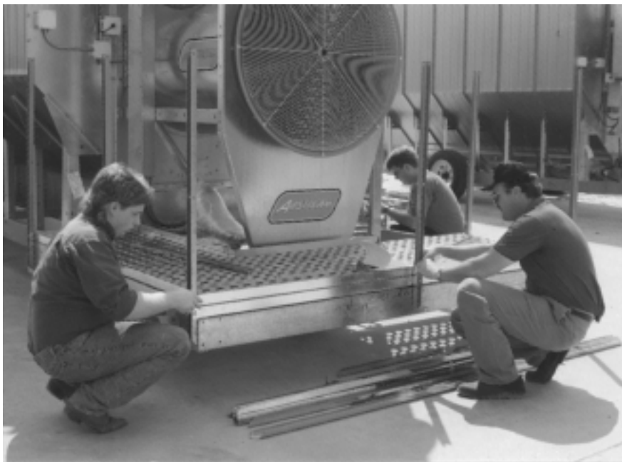
Figure 20: Installing the remaining toe boards.
