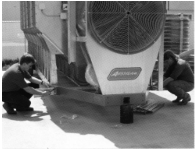
Figure 1, Right: Connecting rear anchor chan- nels. Figure 2, Below: Mount- ing the main support channel.
