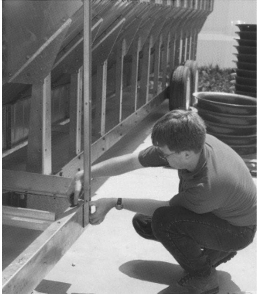
Figure 13: Attaching handrail support channel.
