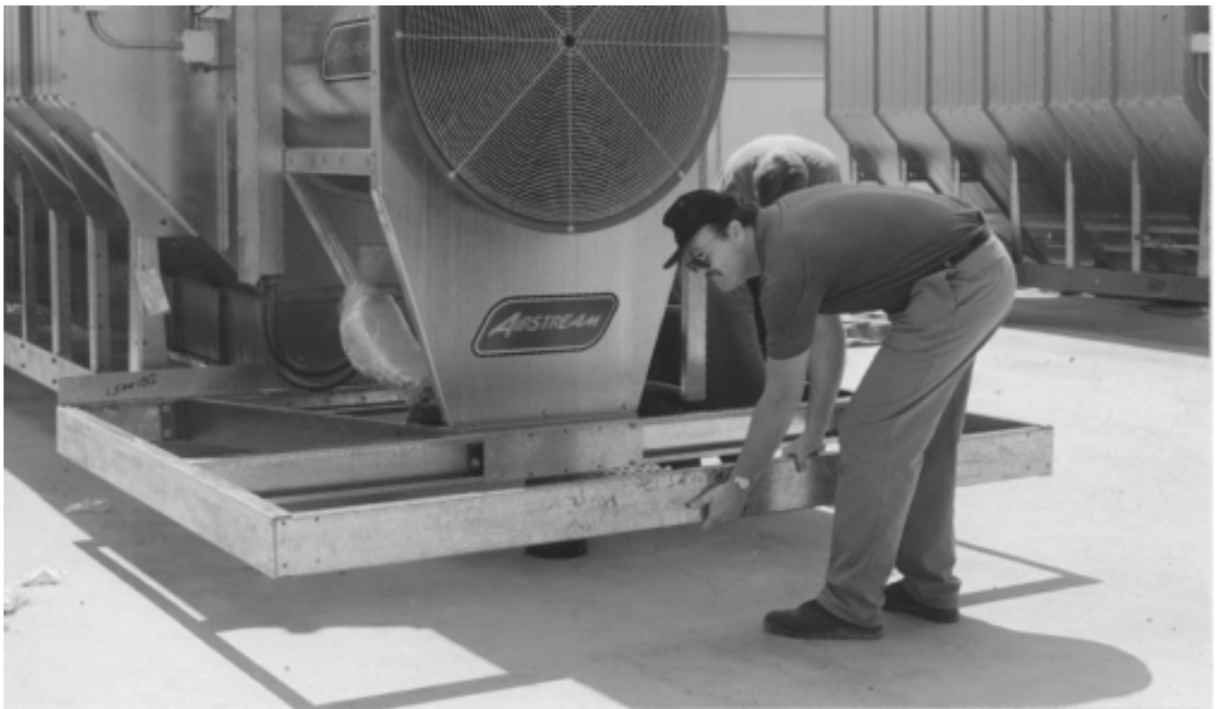
Figure 8: Attaching front channel.
