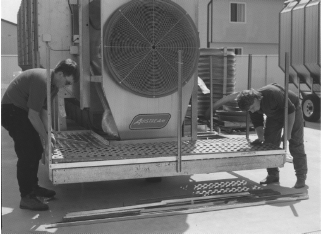
Figure 19: Installing front long floor panel.
