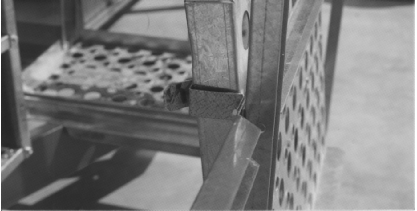
Figure 27: Close-up of access door clip on guard rail.
