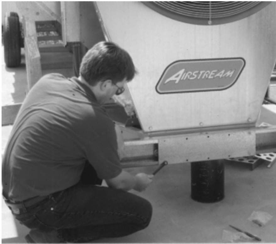
Figure 3: Bolting reinforcement plate to main support channel.
