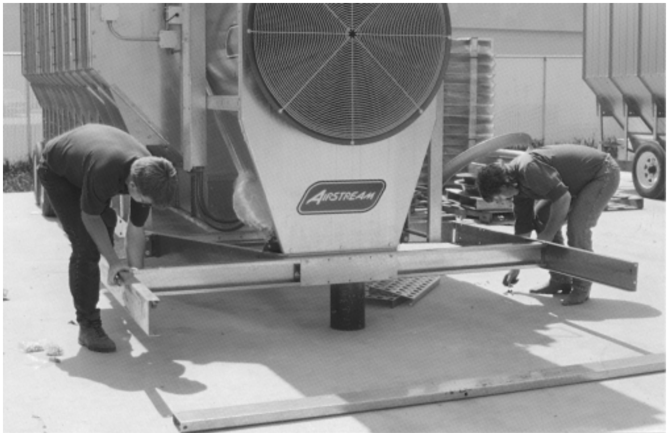
Figure 4: Attaching side channels.
