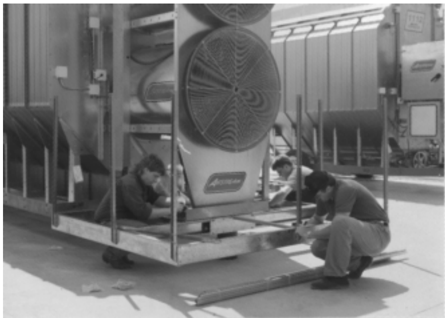
Figure 14: Install remaining support channels.
