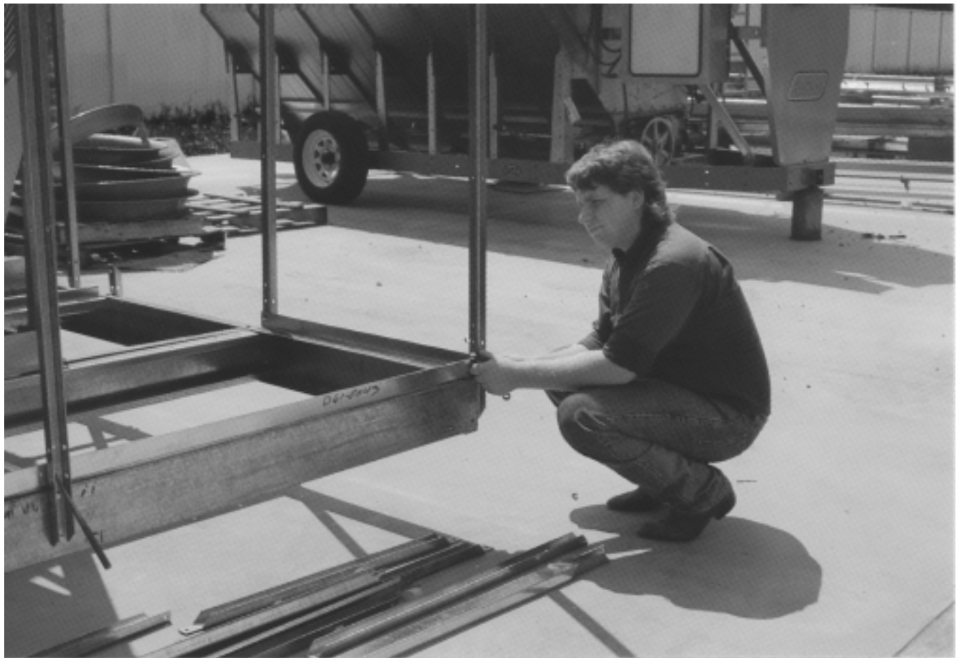
Figure 16: Connecting left-hand front toe board to guard rail support channel.
