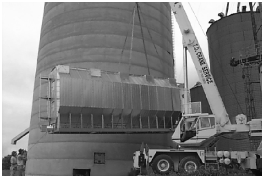
Lifting of 26' Base Module
