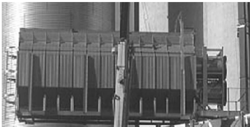
Lifting of 26' Top Module
