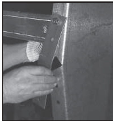
Photo 16-7 Installing RH fan support stiffener with common bolts.
