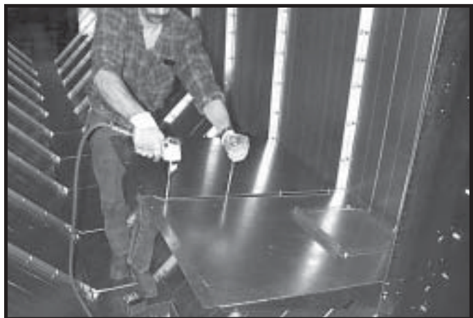
Photo 4-10 Loosely bolting (front) bottom plenum divider overlapping bottom plenum divider end.
