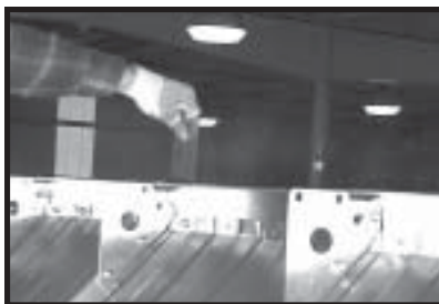
Photo 7-5 Placing top edge angle splice behind top edge angle. (RH side of dryer)
