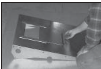
Photo 4-4 Inserting clean-out door between clean-out door guides.
