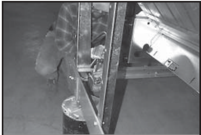
Photo 14-6 Bolting LH side of hitch weldment.
