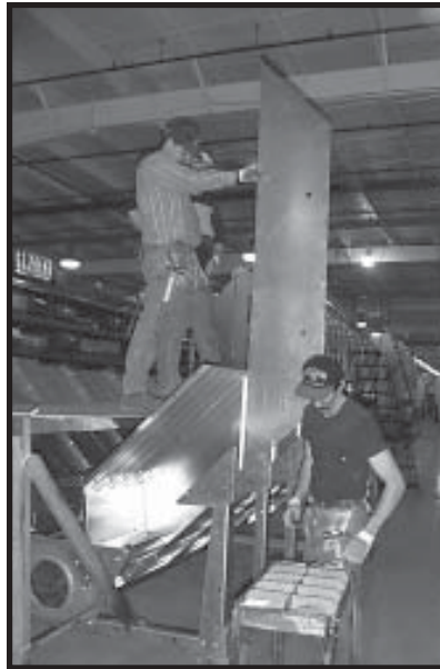
Photo 3-27 Outside-person and inside-person loosely bolt column bulkhead and plenum walls in place.
