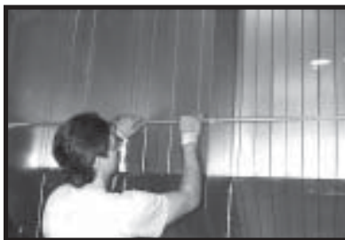
Photo 5-6 Installing connector 1/2” EMT to EMT compression splice in middle of dryer.
