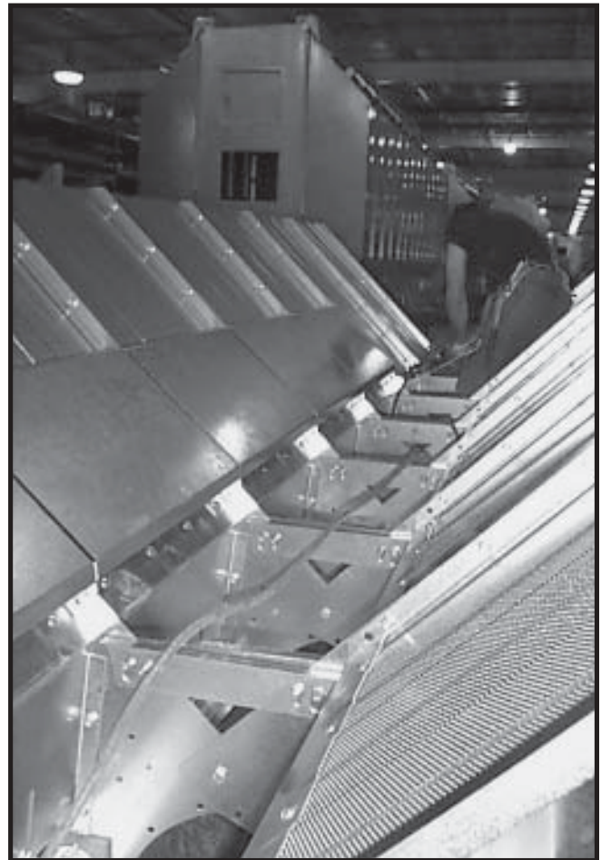
Photo 3-16 Tightening adjusted plenum closure door angles through length of dryer.
