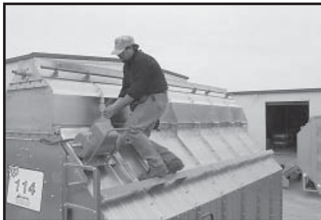
Photo 21-15 Bolting center wet bins to LH wet bin section.
