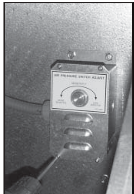
Photo 18-39 Air switch installed.
