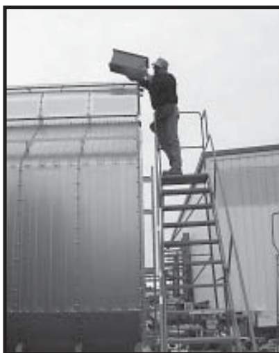
Photo 22-3 Placing hopper assembly (fill).
