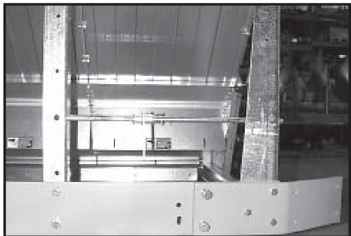
Photo 9-10 Installing pivot rods at front of dryer.
