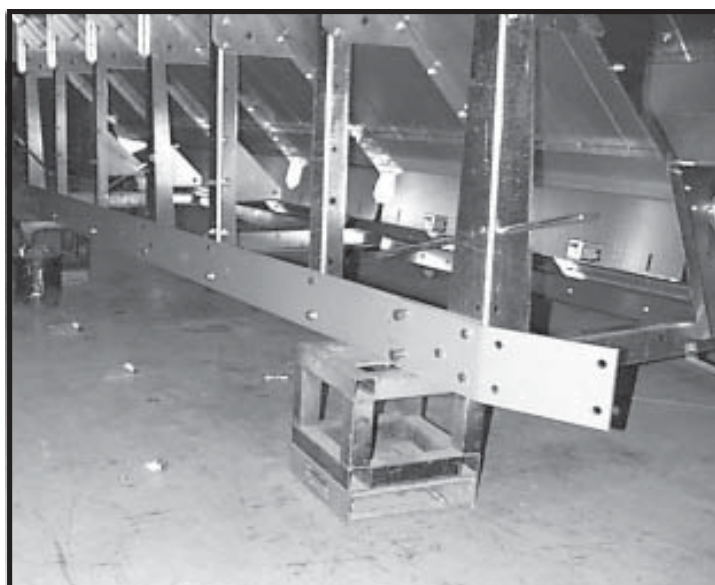
Photo 9-7 Linkage bars and short linkage bar weldments set out by dryer, and pivot rods inserted in pivot rod brackets.
