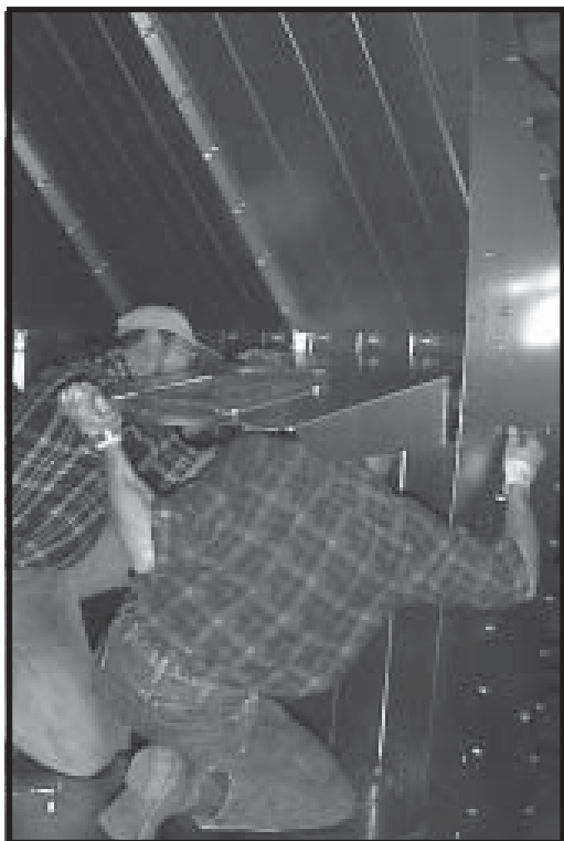
Photo 4-16 Loosely bolting rear edge of (front LH) top plenum divider end to column seam inside dryer.
