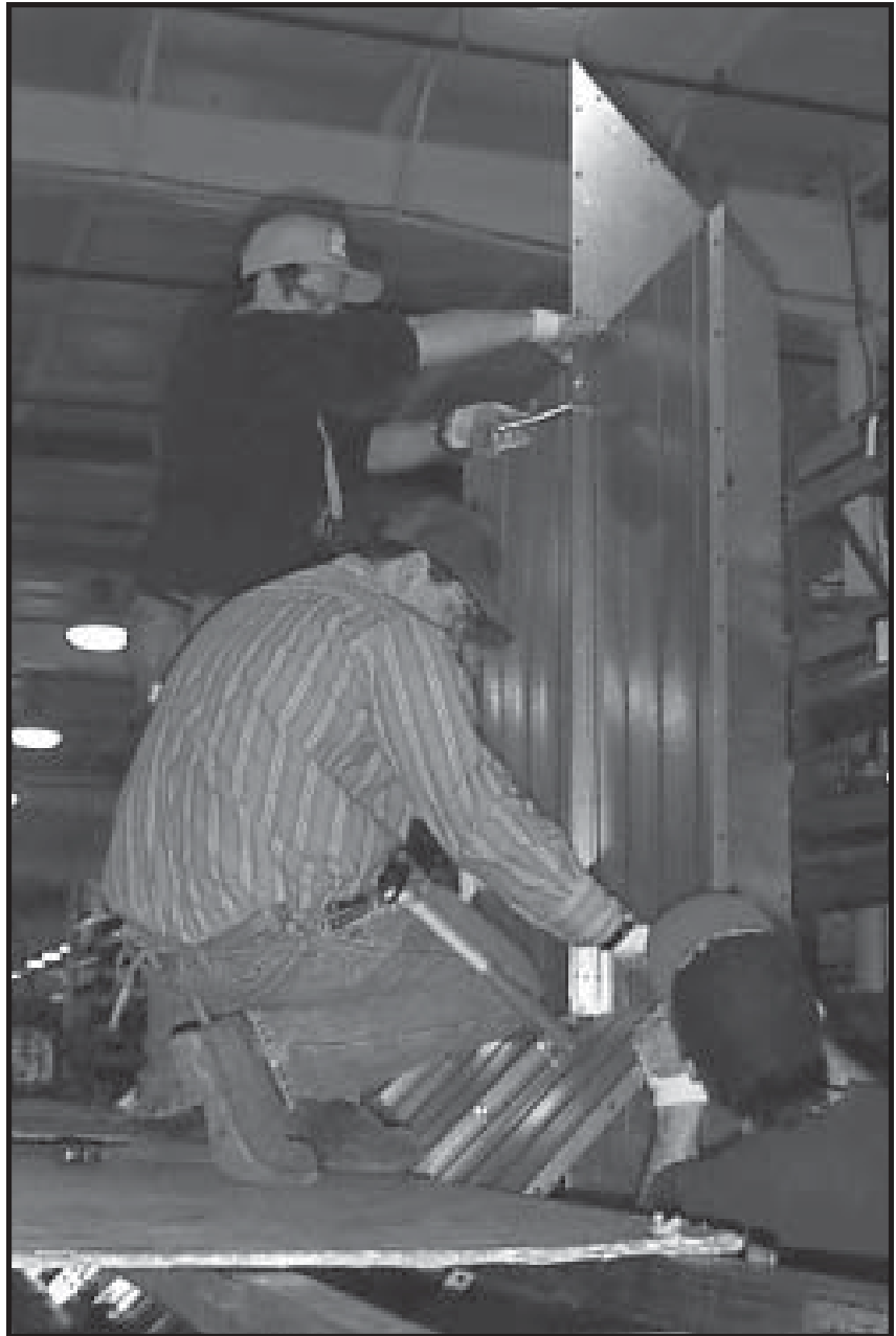
Photo 3-28 Securing first and second PLENUM WALLS on either side of first COLUMN BULKHEAD.
