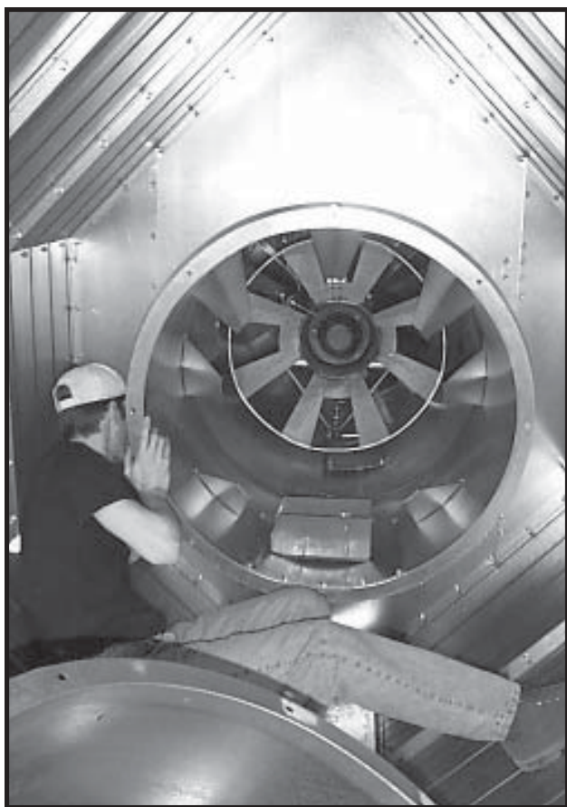
Photo 18-59 View inside dryer - Securing bolts on front airmixer can with nuts inside dryer.
