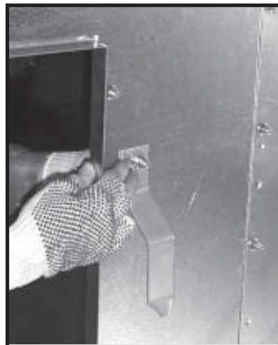
Photo 13-11 Latch bracket installed.
