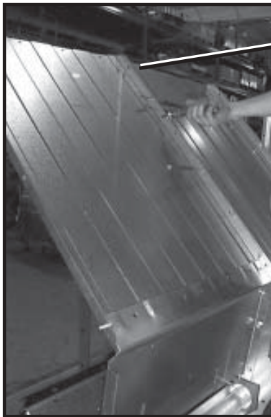
Photo 3-4 Loosely bolting along vertical seams of plenum bottom/hopper bulkhead/plenum bottom .
