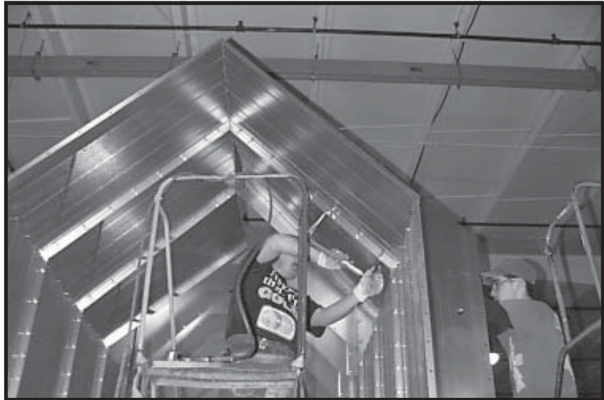
Photo 3-41 Installing plenum tops through length of dryer.
