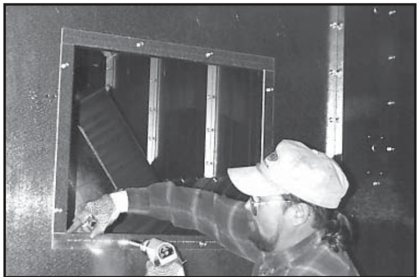
Photo 13-9 Tightening frame for rear door assembly.
