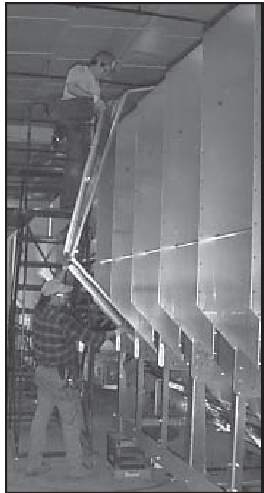
Photo 6-8 Three workers install outside screen pre-assembly consisting of hopper sheet/outside wall/roof sheet.
