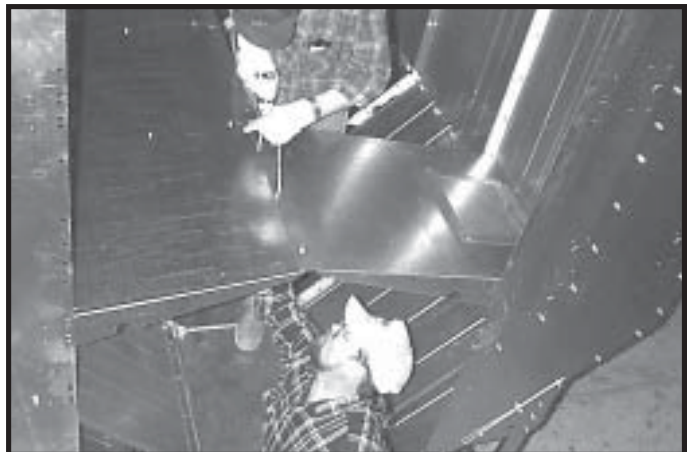
Photo 4-11 Loosely bolting overlapping (rear) bottom plenum dividers.
