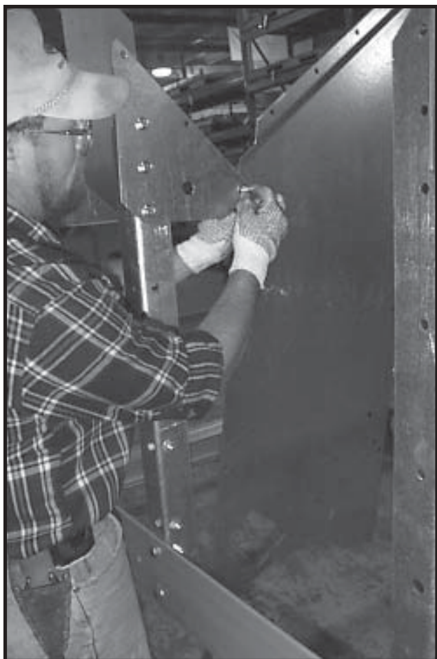
Photo 2-12 Bolting hopper bulkhead to gusset.
