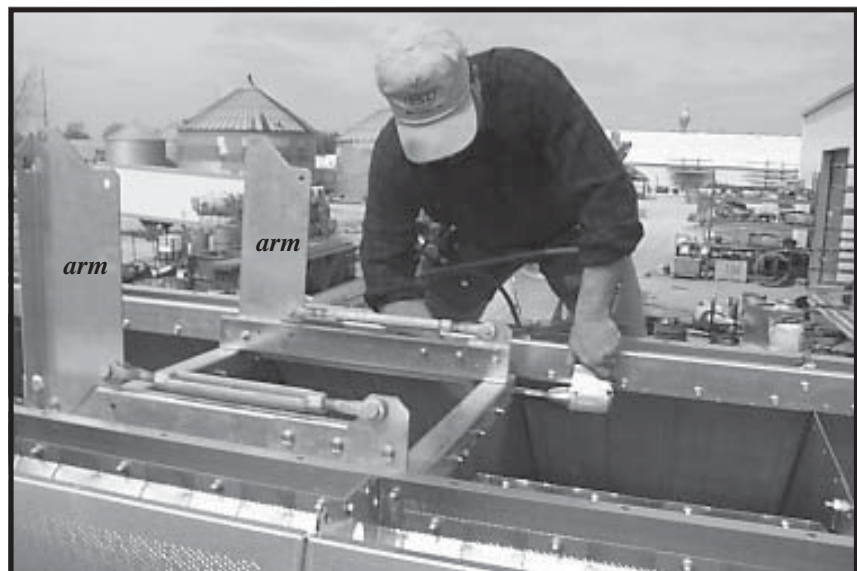
Photo 20-3 Tightening bolts on lift kit. Note lift kit arms are in upright position for installation.
