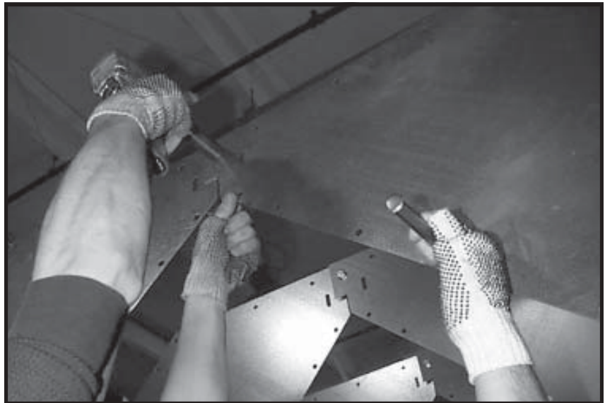
Photo 3-31 Loosely bolting pairs of garner bulkheads through length of dryer.
