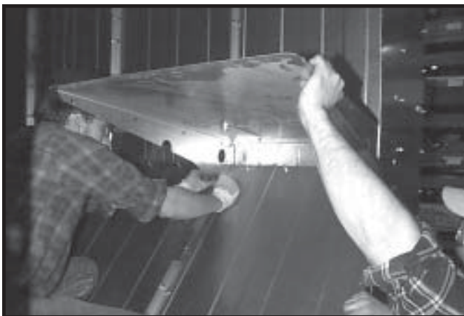
Photo 4-9 Loosely bolting rear edge of (front LH) bottom plenum divider end to column seam inside dryer.
