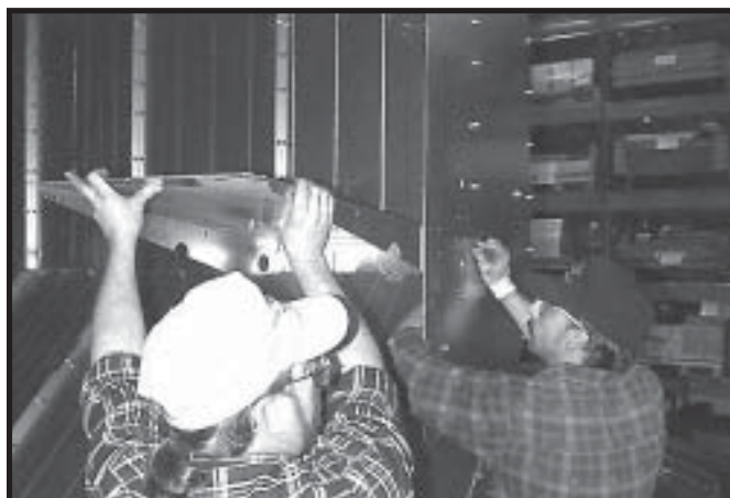
Photo 4-8 Loosely bolting front edge of (front LH) bottom plenum divider end to column end panel.
