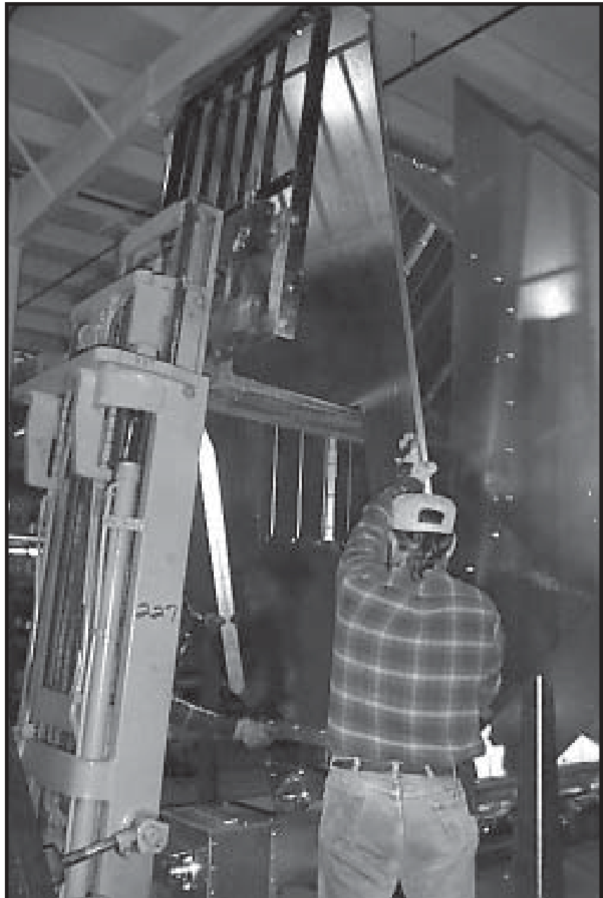
Photo 13-4 Lifting rear end panel onto rear of dryer.
