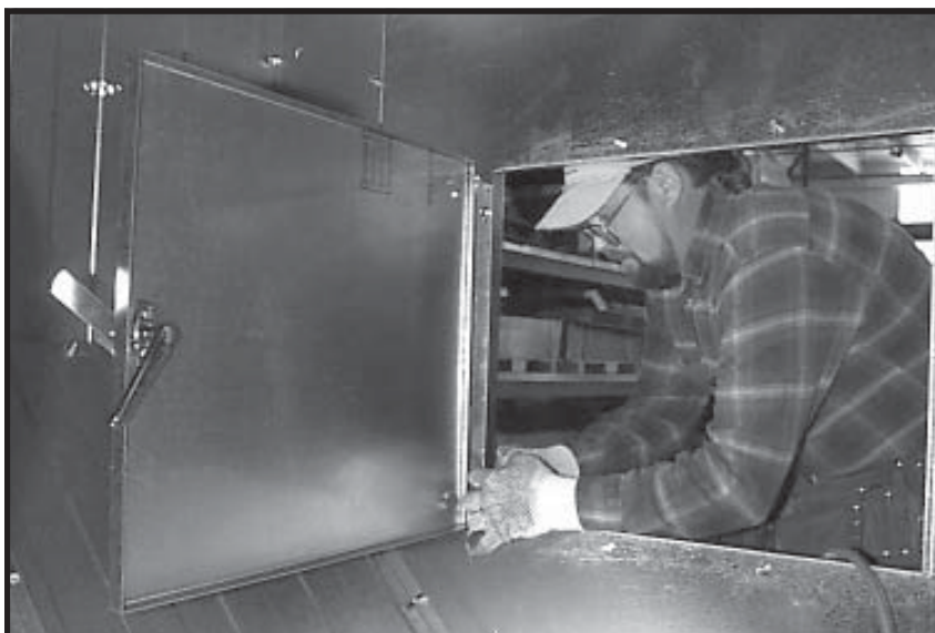
Photo 13-12 Installing rear door assembly.
