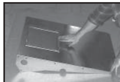
Photo 4-5 Checking clean-out door.
