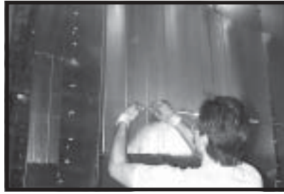
Photo 5-8 Installing connector 1/2" EMT compression (without locknut) at front of dryer.
