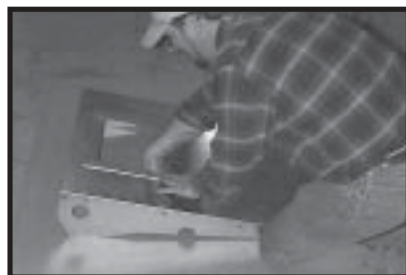
Photo 4-3 Bolting clean-out door guides to bottom plenum divider end.
