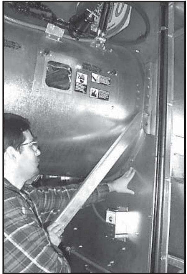
Photo 18-61 Front diagonal support channel bolted to diagonal support bracket.
