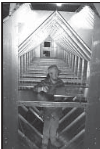
Photo 4-24 Placing first pair of plenum sheets. (rear view)
