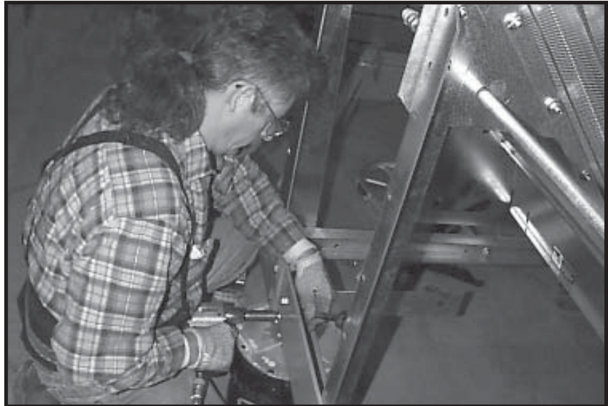
Photo 15-6 Tightening motor mount support bracket (for SCR motor).
