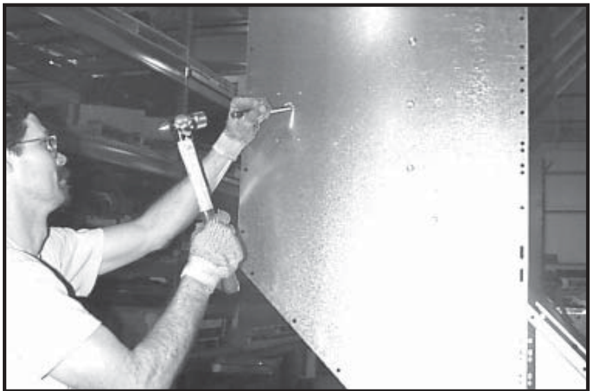
Photo 3-44 Removing knockout in column end panel.
