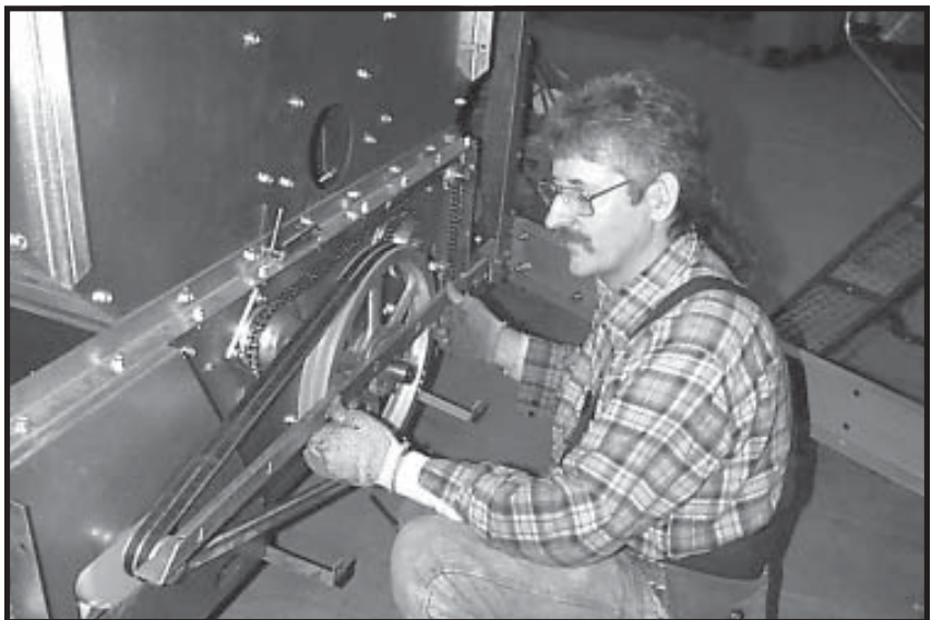
Photo 15-21 Aligning belts across pullies with straight edge.
