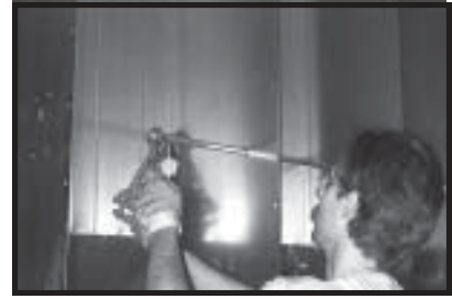
Photo 5-9 Tightening connector 1/2" EMT compression at front of dryer.
