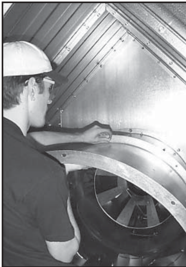
Photo 18-60 View inside dryer - Securing bolts on front airmixer can with nuts inside dryer.
