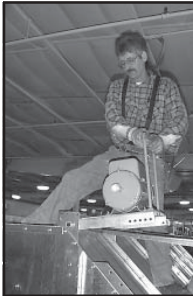
Photo 15-25 Installing load motor.
