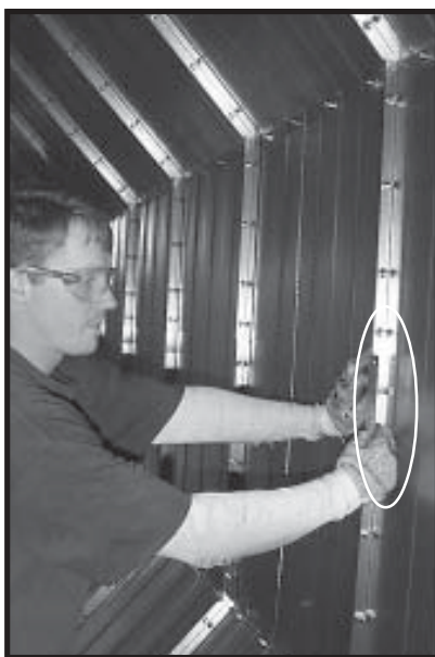
Photo 12-12 Close up - installing capillary brackets.
