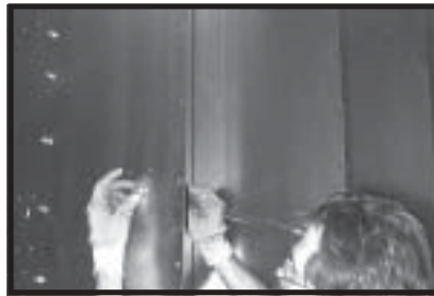
Photo 5-10 Installing locknut.
