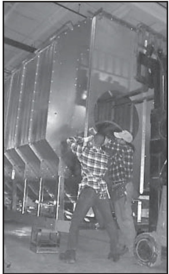
Photo 12-9 Loosely bolting front end panel to column end panel up to about six feet.
