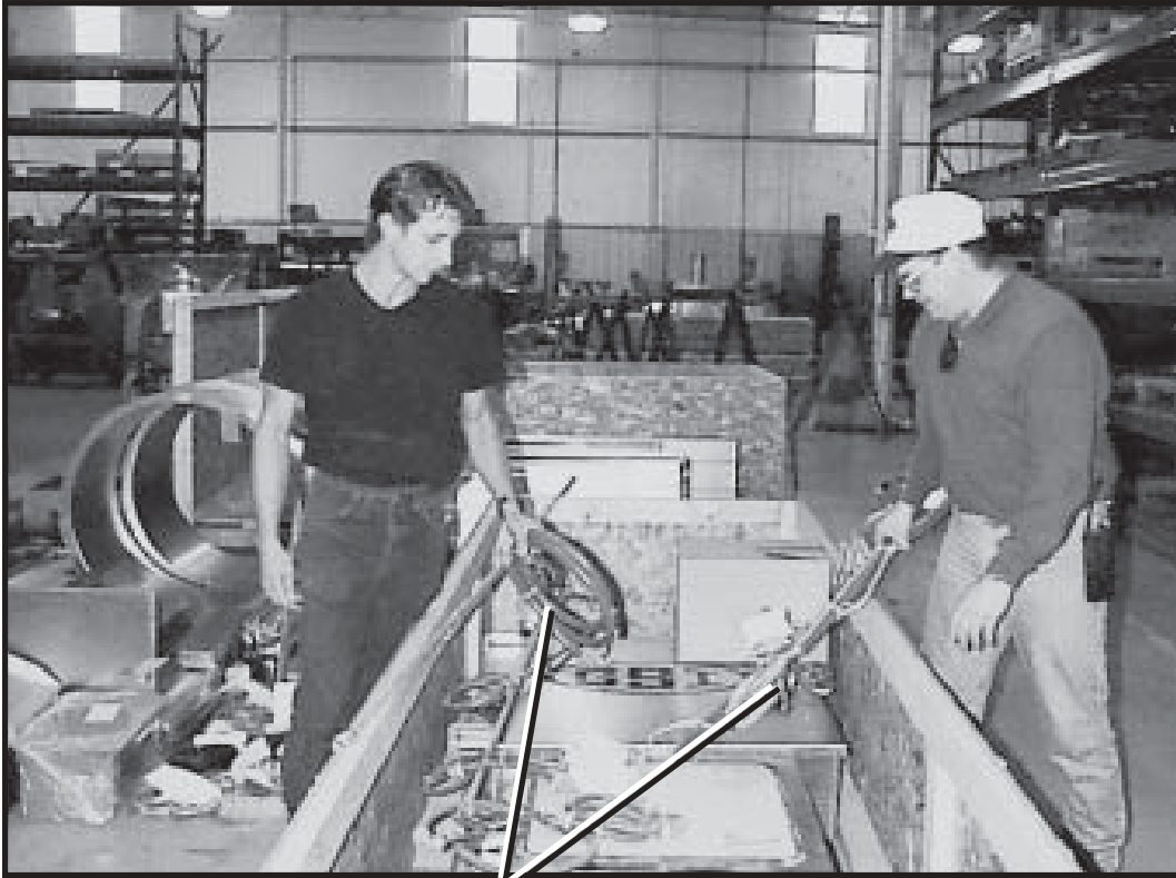
Photo 1-11 Unpacking electrical conduit assemblies from control box crate.
