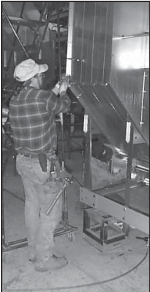
Photo 6-9 Close Up - Outside screen installation.
