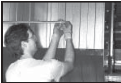
Photo 5-4 Installing connector 1/2” EMT compression at rear of dryer.
