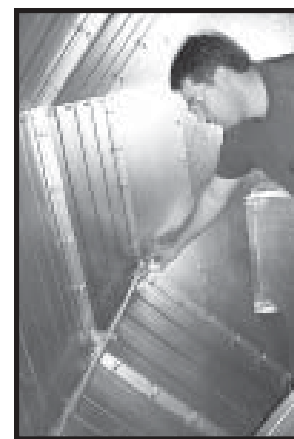
Photo 18-6 Thermister installed on plenum pipe inside rear of Series 2000 dryer.
