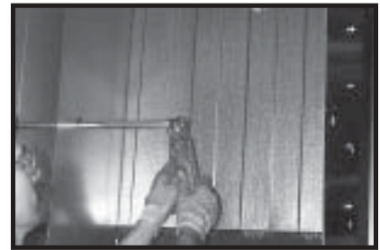
Photo 5-5 Tightening connector 1/2” EMT compression at rear of dryer.
