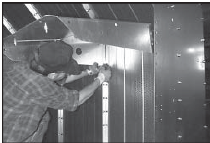
Photo 4-17 Loosely bolting front edge of (front LH) top plenum divider end to column end panel.
