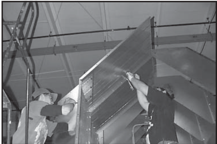
Photo 3-34 Close up - Positioning second plenum top to rear of garner bulkhead with 3/8" punches, securing with clamps, and loosely bolting.
