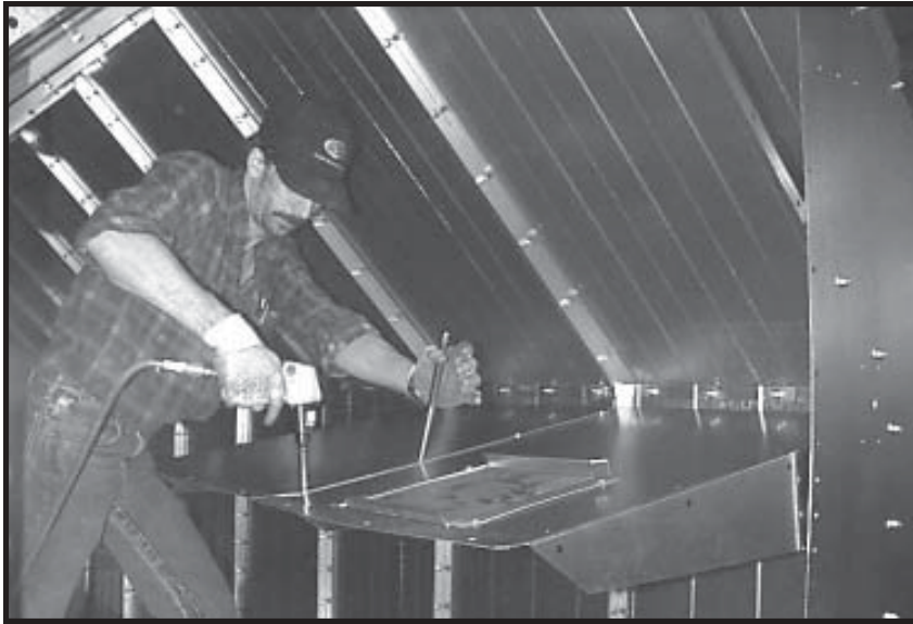
Photo 4-18 Tightening screws in (front) top plenum divider overlapping (front LH) top plenum divider end.
