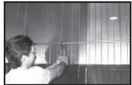
Photo 5-7 Tightening connector 1/2” EMT to EMT compression splice in middle of dryer.
