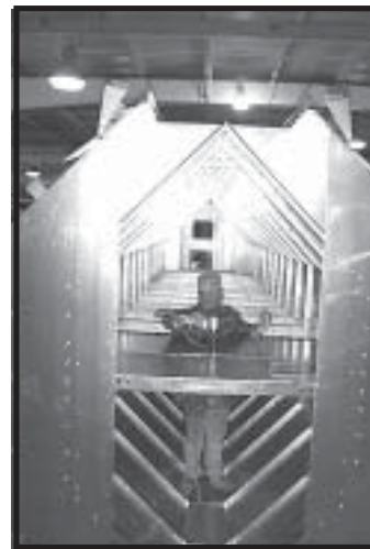
Photo 4-25 Loosely installing screws in next pair of plenum sheets.
