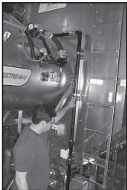
Photo 18-67 NG Pipetrain installed.
