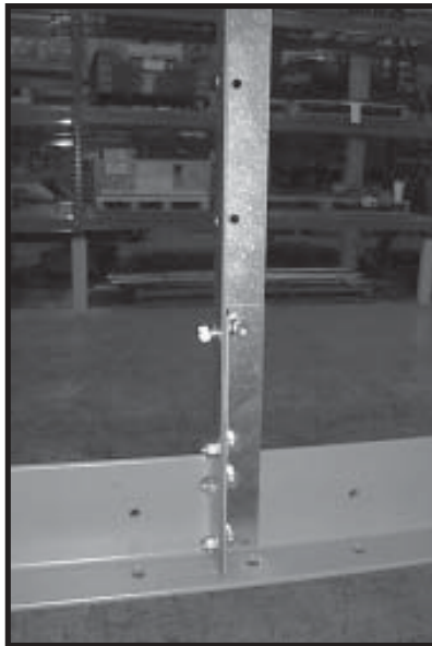
Photo 2-4 Loosely bolt stiffner angle.
