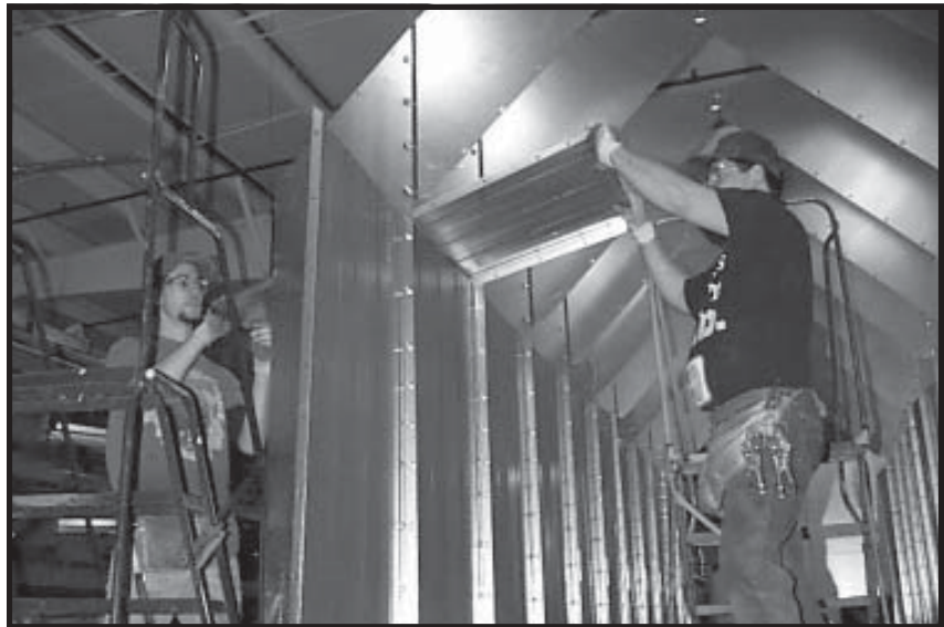
Photo 3-33 Outside-person lifting first plenum top up to inside-person.
