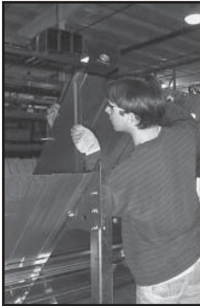
Photo 3-3 Outside-person lifts plenum bottom into place, inside-person bolts it.
