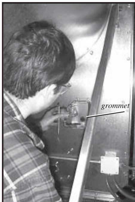
Photo 18-38 Wiring air switch.
