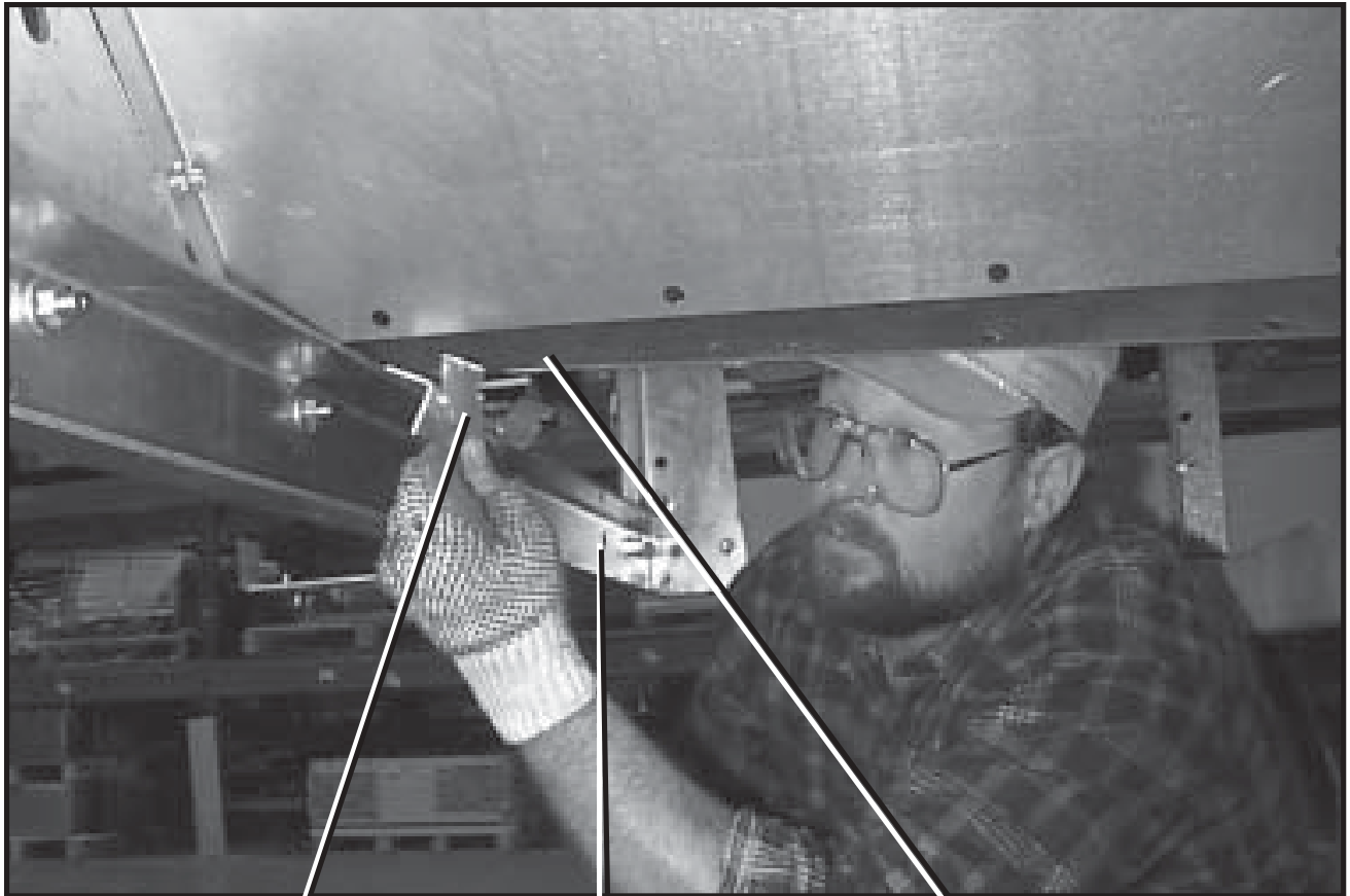
Photo 2-24 Place end seal on top of frame tie channel and on outside of trough panel.
