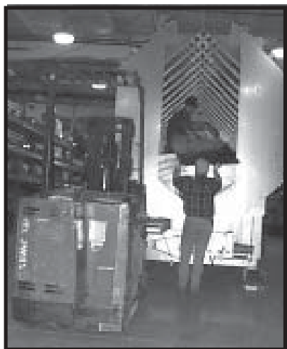
Photo 4-15 Lifting top plenum dividers up for installation.
