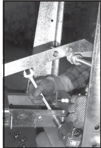
Photo 15-17 Installing motor mount adjustment bracket to motor mount support bracket.
