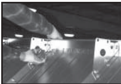
Photo 7-6 Bolting top edge angle splice. (RH side of dryer)
