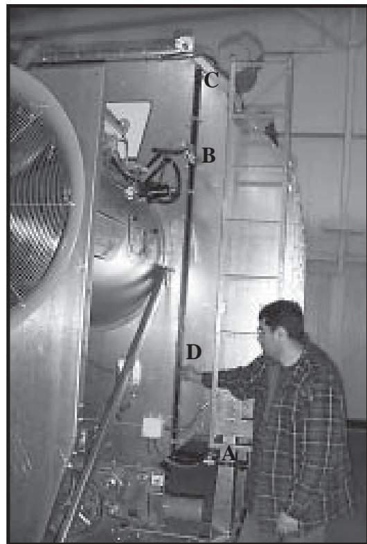
Photo 18-65 Example - LP Pipetrain installed to Series 2000, 10' dryer.
