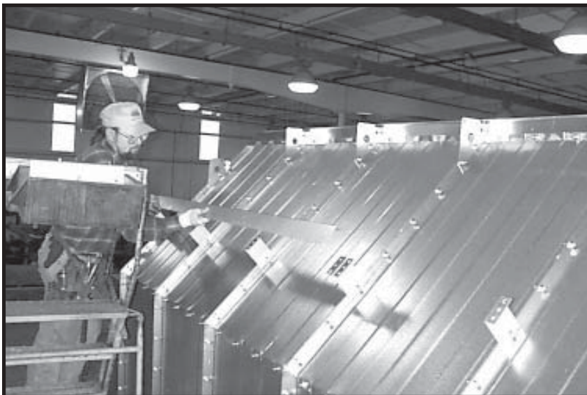
Photo 7-12 Placing top edge angle over walk rail brackets. (RH side of dryer)
