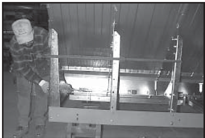
Photo 9-11 Installing pivot rods at rear of dryer.
