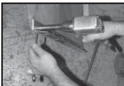
Photo 12-5 Bolting top angle bracket to top of front end panel.
