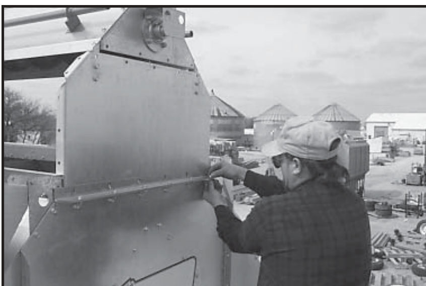
Photo 21-12 Rear view - installing top edge angle.
