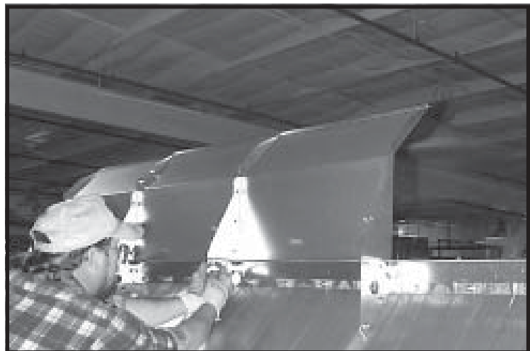
Photo 17-4 Use 5/16"x3/4" whiz bolts and nuts at pivot points.
