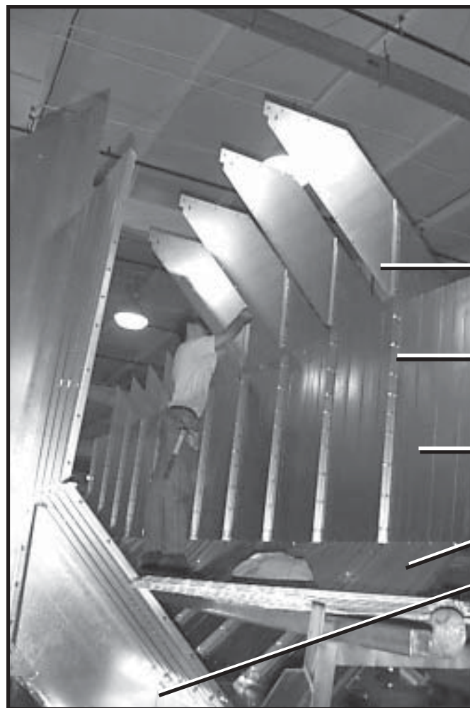
Photo 3-30 Loosely bolting garner bulkhead to column bulkheads through length of dryer.
