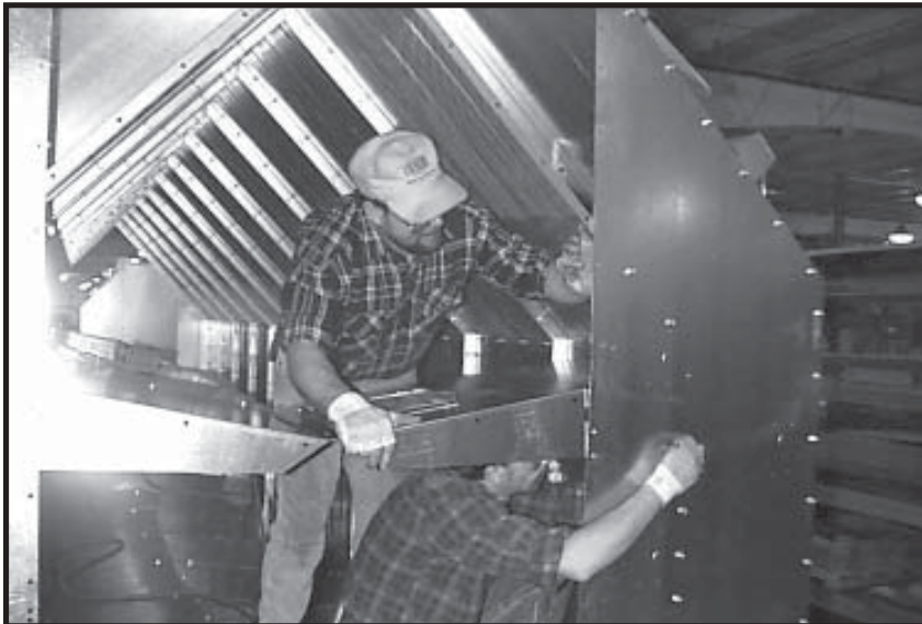
Photo 4-19 Installing (rear RH) top plenum bottom end.
