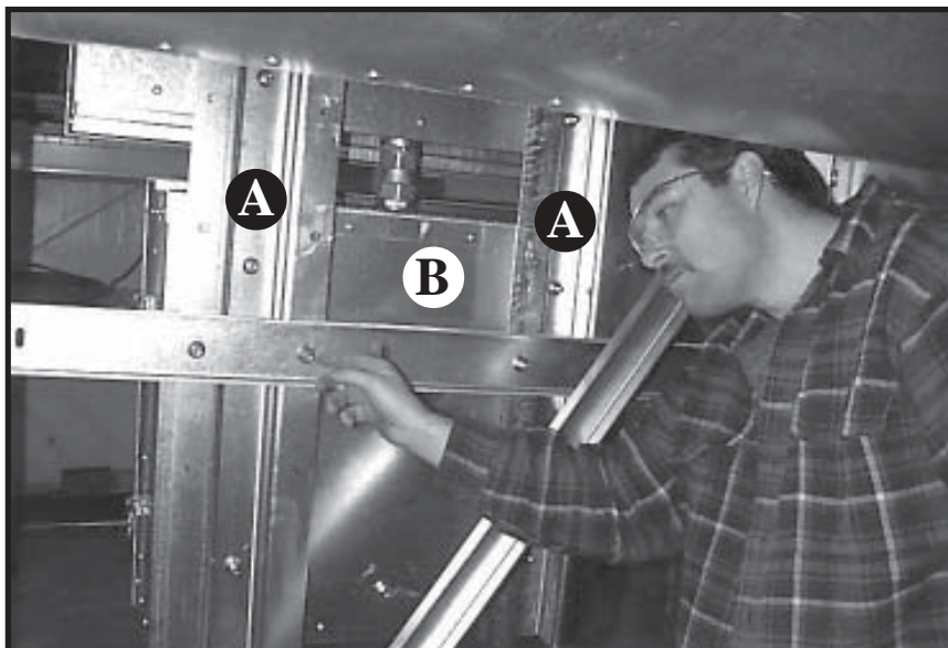
Photo 18-76 Inside view - (2) control panel supports (A) (with control box (B) already installed).
