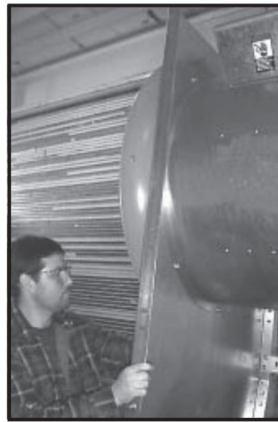
Photo 18-57 Rear view - Venturi loosely bolted with common bolts through front fan support to fan-heater assembly.
