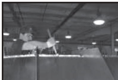
Photo 3-39 Hammering gaps closed.
