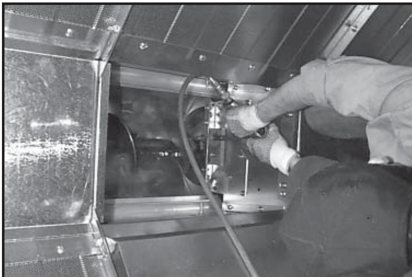
Photo 3-21 Tightening hanger bearing assembly to C-channel mount.
