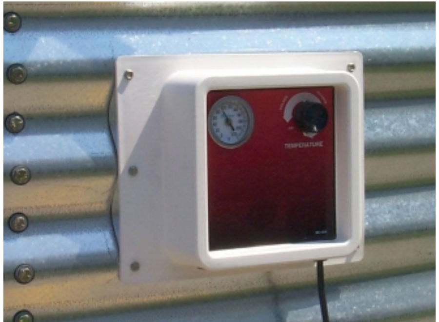
Plenum thermostat mounted on bin wall.
