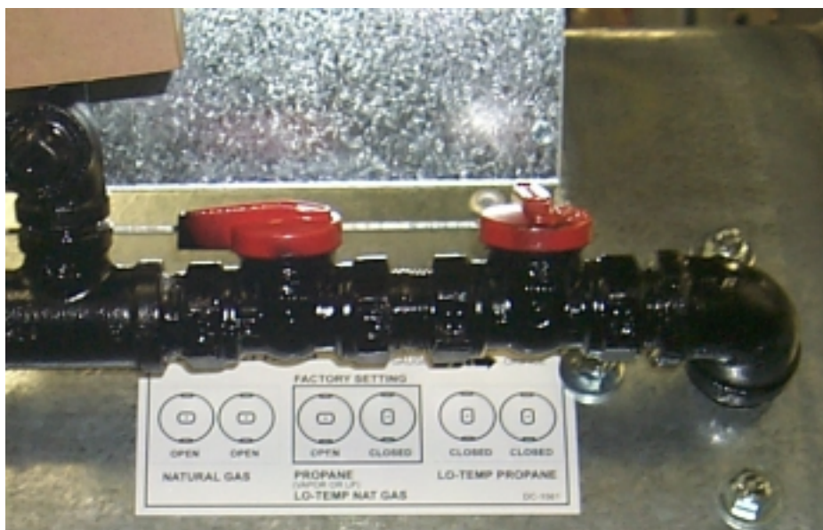
Orifice Valves installed on heater and configured for Propane.
