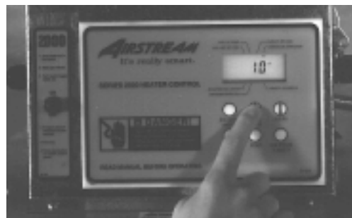
Programming the temperature differential.
